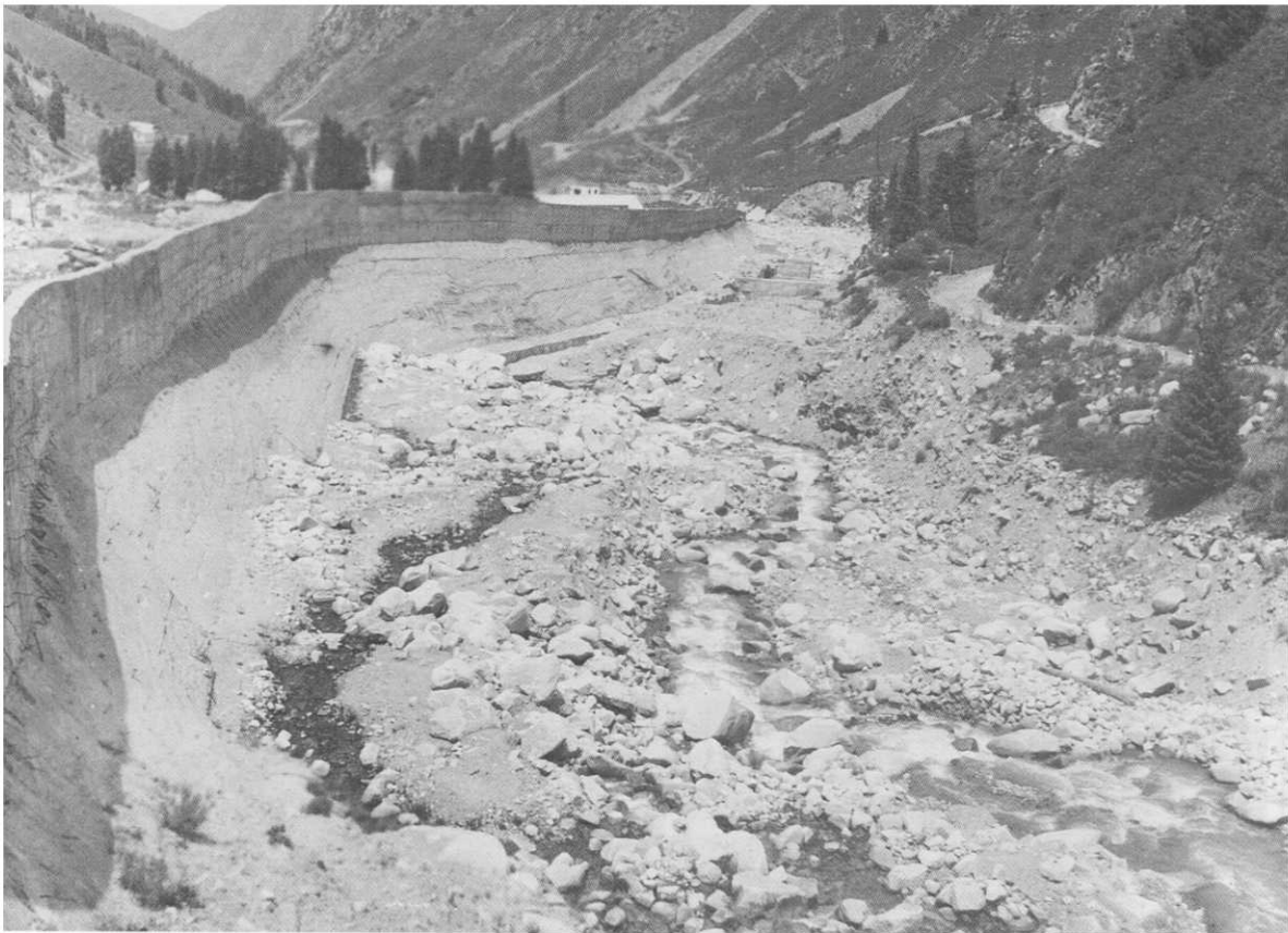
FIGURE 8.49 (c) (ii) Mudflow protection wall on the Bolshaya Almatinka River constructed after the mudflow disaster of 1977.
