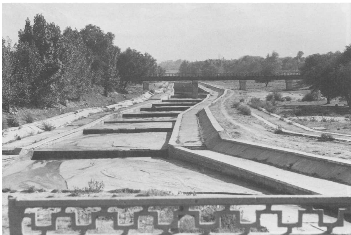
FIGURE 8.49 (c) (i) Flow stabilization structure on Bolshaya Almatinka River.
