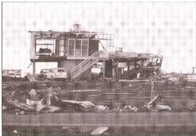
Figure 6: Damage to elevated house following Cyclone Tracy, Darwin, 1974
