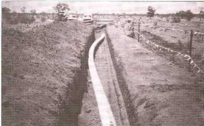
Figure 3: The impact of the Tennant Creek earthquake, 1988 a Ground rupture b A warped gas pipeline
