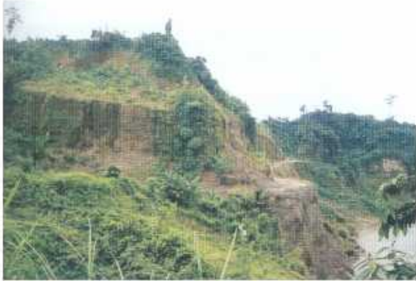
Sinking of hill and the road - Arunachal Pradesh
