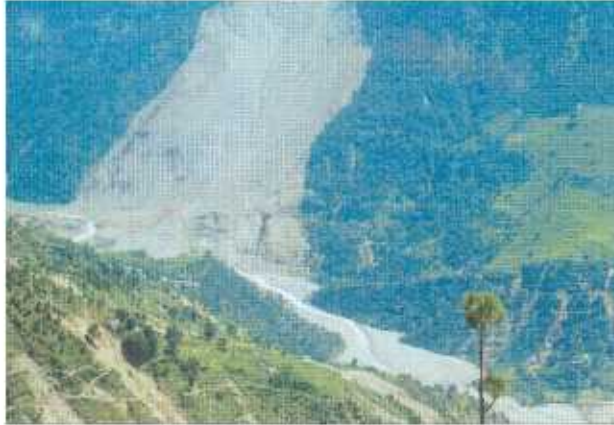
Dokhimat Landslide (1998) - Uttar Pradesh
