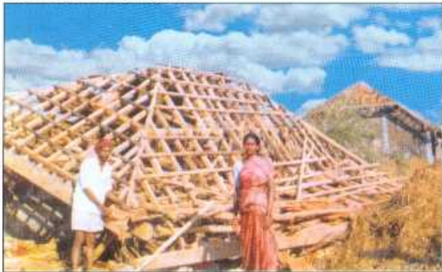
Gadimaga Village, East Godavari District : Damage caused due to cyclone
