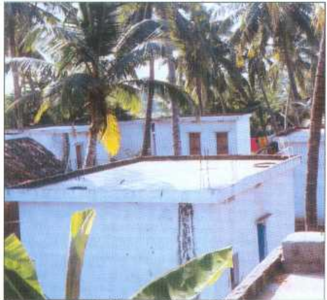
Madhavarayudupeta Village, East Godavari District. Permanent houses constructed with cyclone resistant features
