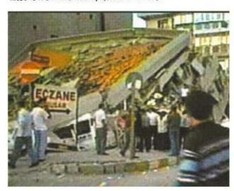
images of destruction in Turkey confirmed what seismic engineers already knew, that a powerful eqrthquake has an ally in a weak building.
