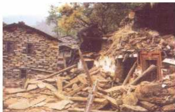
Non-engineered building collapsed due to earthquake in Chamoli
