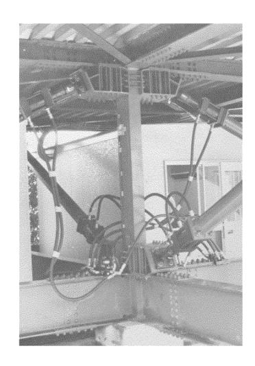
Fig. 2.7 Joint Configuration of Active Brace
