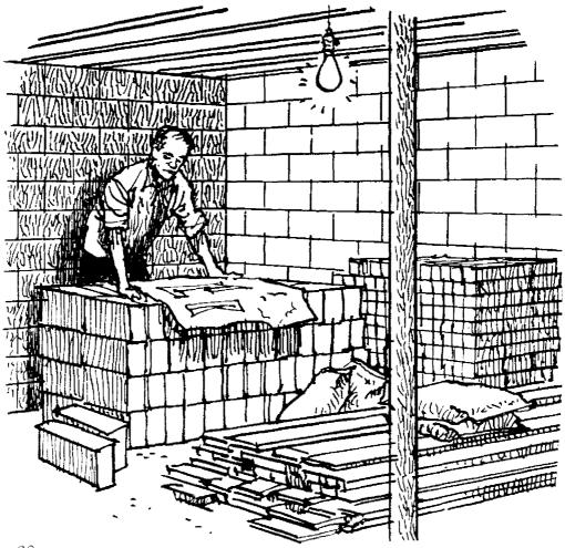
◆ A PERMANENT BASEMENT SHELTER. If your home basement for one corner of it—is below ground level, your best and easiest action would be to prepare a permanent-type family shelter there. If you have basic carpentry or masonry skills, you probably could buy the necessary shielding material and do the work yourself in a short time.
