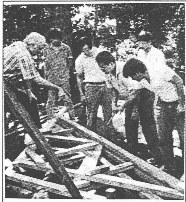
Figure 2.2.1 Community participation is the only viable route for people in solving their housing problems in developing countries.
