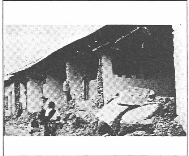
Figure 6.1-3 A substantial percentage of the population of Chimaltenango, Guatemala, died in their heavy-walled adobe buildings. East Anatolian and Iranian adobe buildings are even deadlier, because of their heavy roofs of tree trunks or rafters topped with a thick earth cover.
