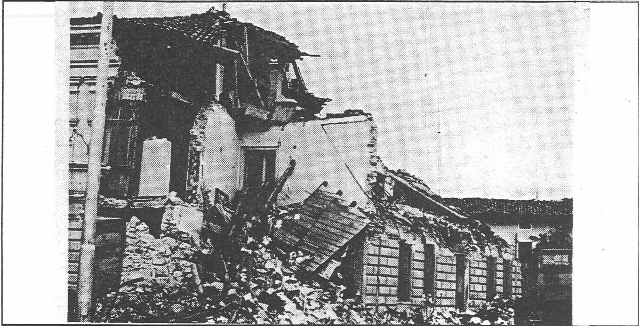
Figure 13.1-9a Collapsed brick buildings at Osoppo, Friuli, Italy. This M 6.5 event caused very severe losses to brick buildings. An old lesson was repeated, viz. that brick is not suitable for structural elements in earthquake zones.
