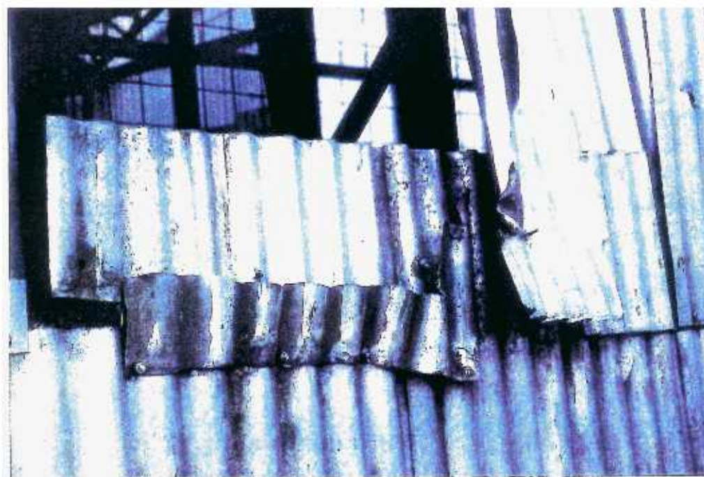
14 Friars Hill Workshop - note the torn corrugated steel sheets
