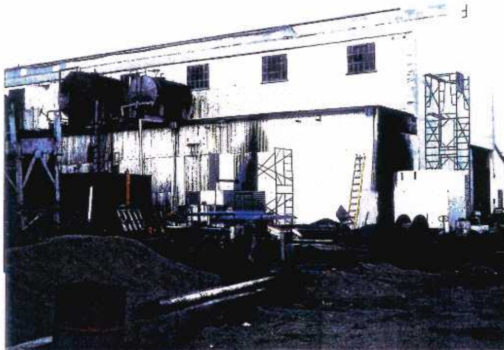
8 Friars Hill Power Station - the south gable-end cladding has been replaced since the hurricane.
