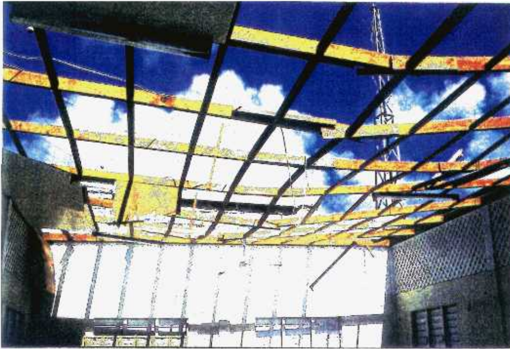
5 Cassada Gardens Canteen - roof structure completely removed; ceiling structure badly damaged, but in place.
