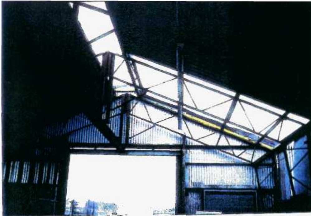
16 Friars Hill Workshop - view from inside showing loss of gable-end and ridge sheeting
