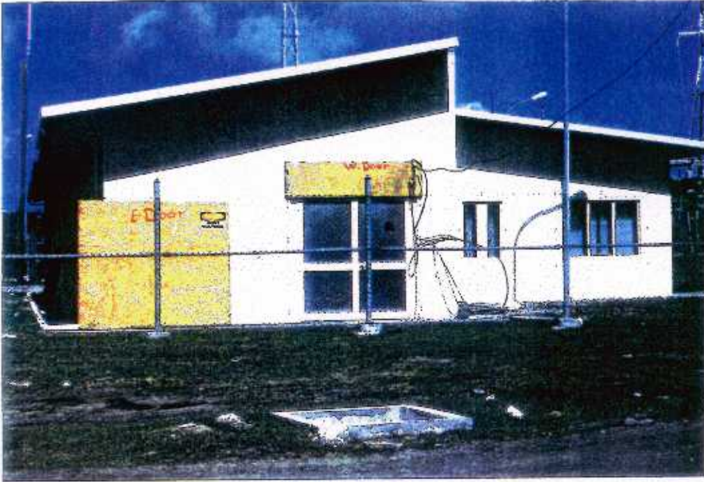
27 Cassada Gardens Complex - hurricane shutters were in place during Luis
