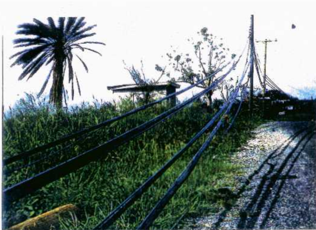
56 Many of the poles were overloaded with telephone and television cables (Jonas Road)
