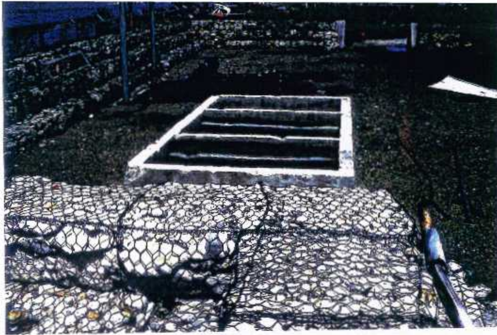
41 Crabbs Complex - gabion cofferdam protecting equipment pit outside of Diesel Power Station (note gap in the wall)
