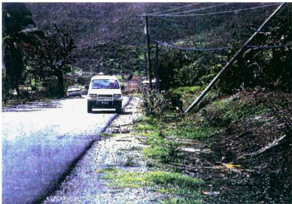
52 The leaning poles were planted before the road was excavated (west of Old Road). This led to less eventual foundation depth than was intended.
