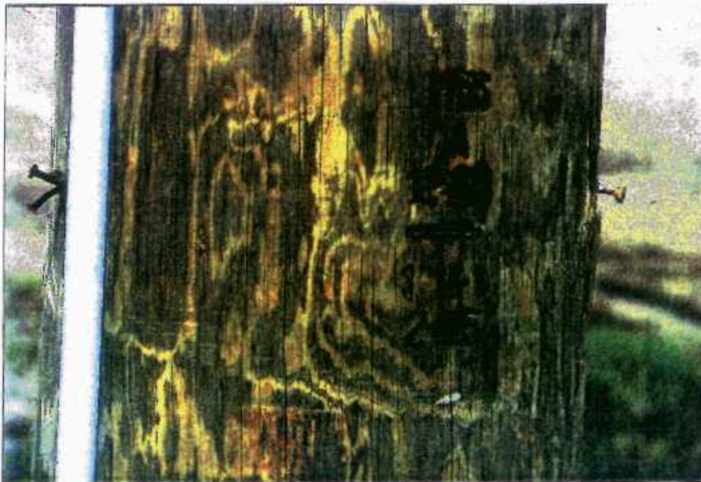
50 Poles are marked with manufacturer's recommendations for embedment
