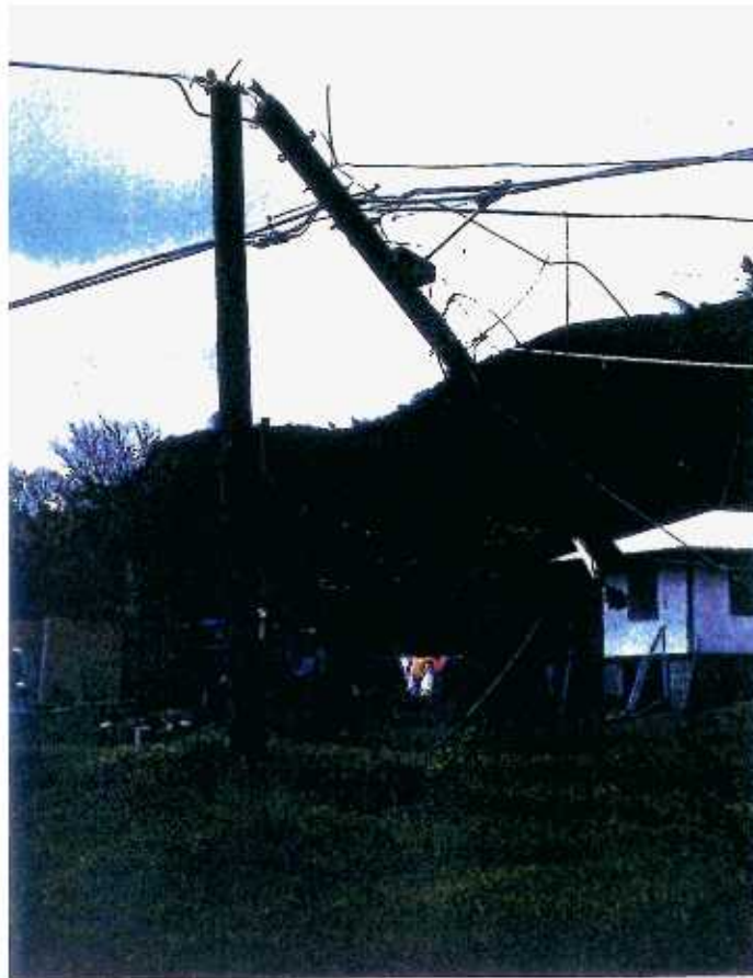
53 The pole broke at the location of a drilled-through tie anchorage
