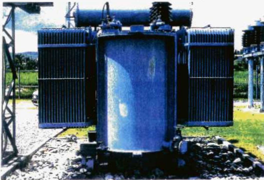
59 Heavy equipment may not be vulnerable in hurricanes, but need to be anchored for the earthquake hazard.
