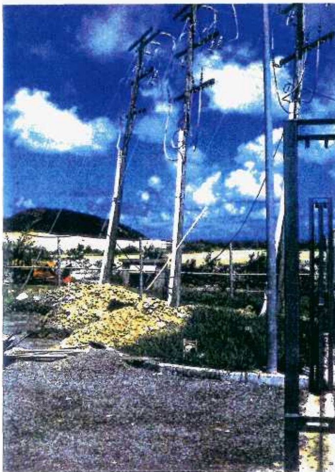
51 End of the line at Five Islands Substation - note the leaning poles indicating incipient failure of the anchorages
