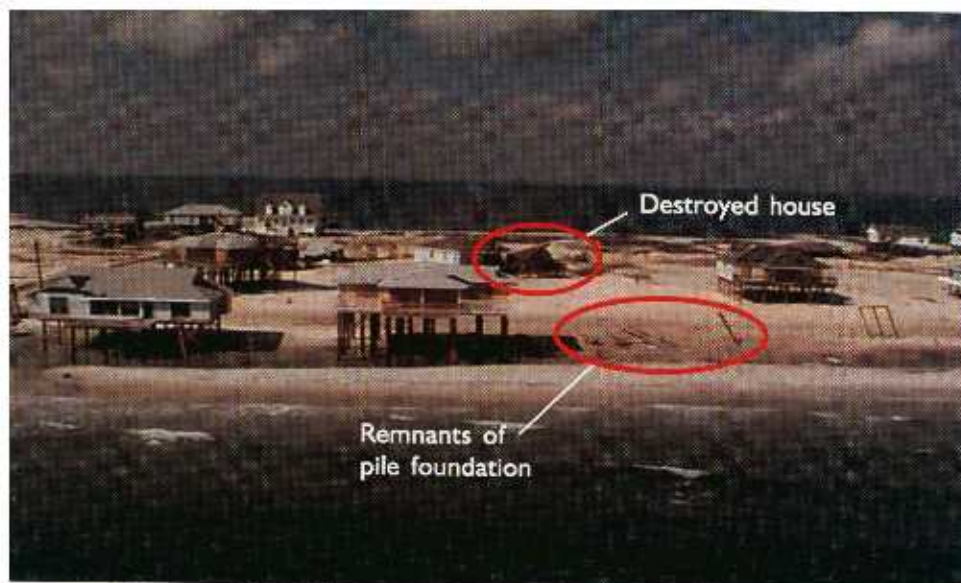
FIGURE 3-4 Front-row house separated from its foundation and destroyed by the storm on Dauphin Island, Alabama. Note the properly elevated and set back house on the right fared very well.
