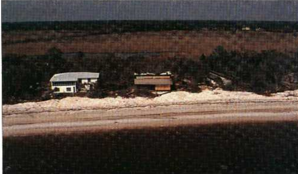
FIGURE 3-6 Overwashed sand accumulation and minor structural damage near Gautier, Mississippi.
