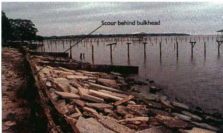
FIGURE 3-7 Remnants of fishing piers in Mobile Bay near Fairhope, Alabama. Note scour behind the bulkhead on the left.
