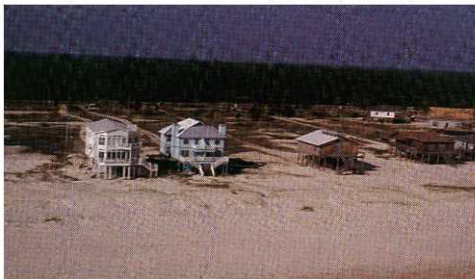
FIGURE 3-10 Properly elevated and set back houses sustained little damage.
