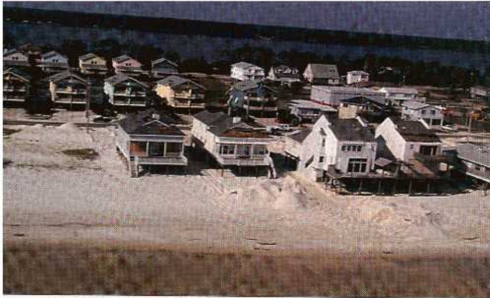
FIGURE 4-36 Houses in Gulf Shores with roof damage. Note loss of roof covering on front-row buildings.
