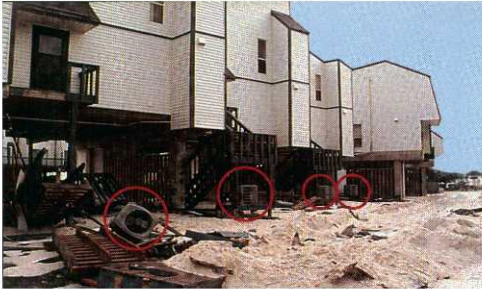
FIGURE 4-23 These air conditioner/heat pump compressors in Gulf Shores were not elevated and therefore were severely damaged.
