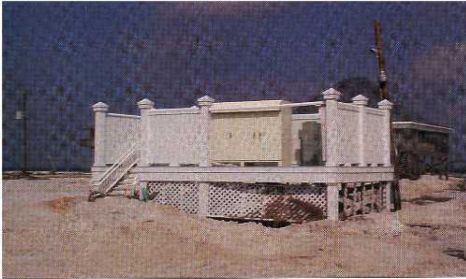
FIGURE 4-20 Other than losing part of the lattice screening, this elevated utility platform performed well.
