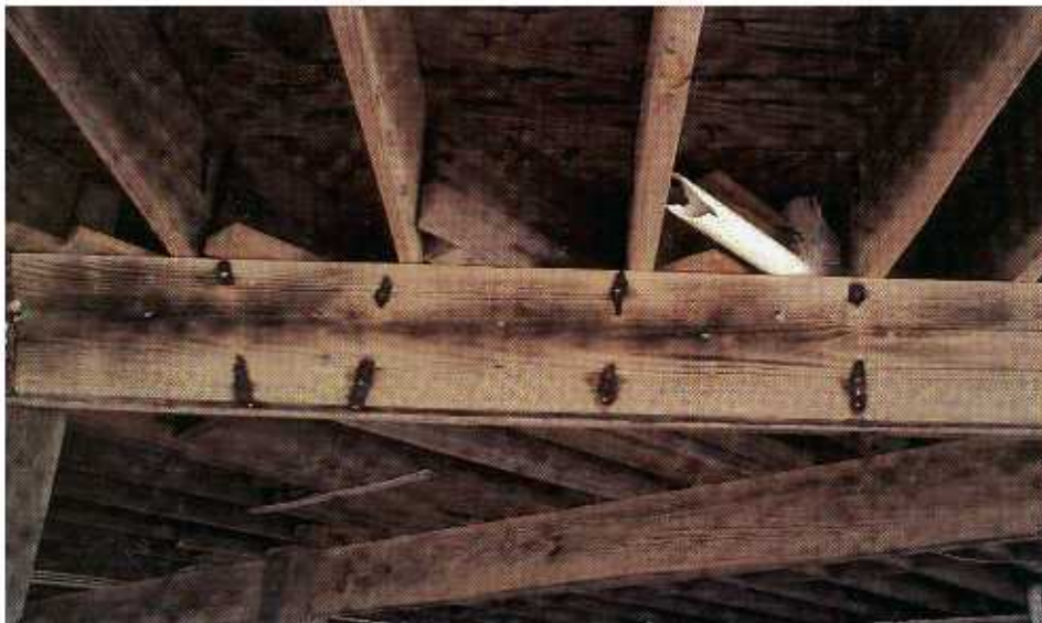
FIGURE 4-24 Only remnants of corroded hurricane straps remain.
