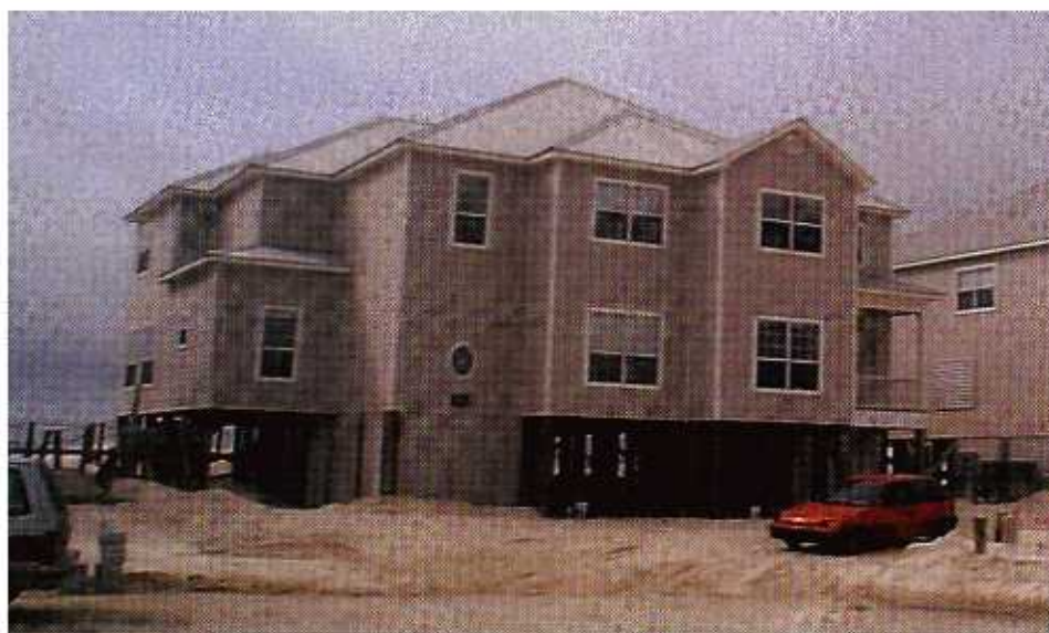
FIGURE 4-39 Fiber-reinforced concrete siding suffered no damage.
