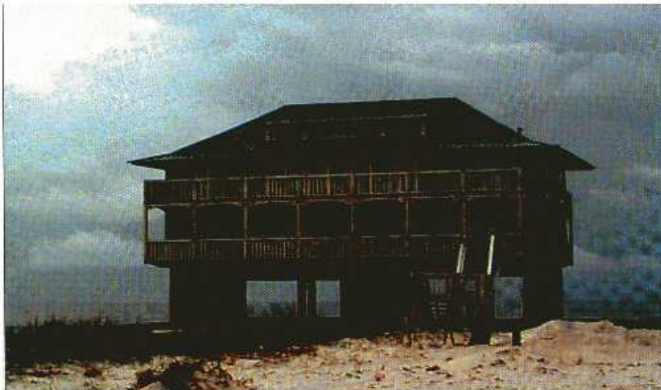
FIGURE 4-27 This properly elevated structure in Gulf Shores suffered no damage other than the loss of breakaway walls and slight damage to its stairs.
