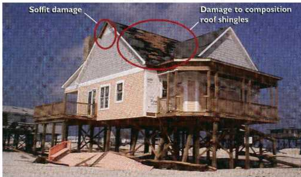
FIGURE 4-34 Wind damage to composition roof shingles and siding on newly built coastal home.
