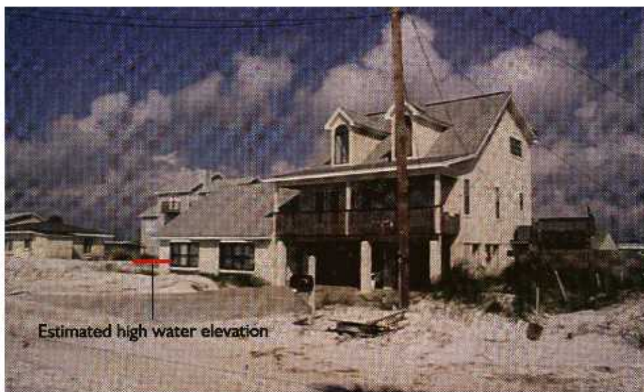
FIGURE 5-10 An existing slab-on-grade home was expanded with a properly elevated addition.
