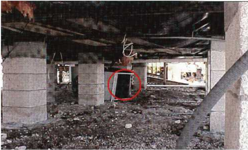
FIGURE 5-18 Reinforced masonry pier foundation system under a newer manufactured home that performed well. The air conditioner compressor (circled) washed under the home provides evidence of the coastal surge at this location.
