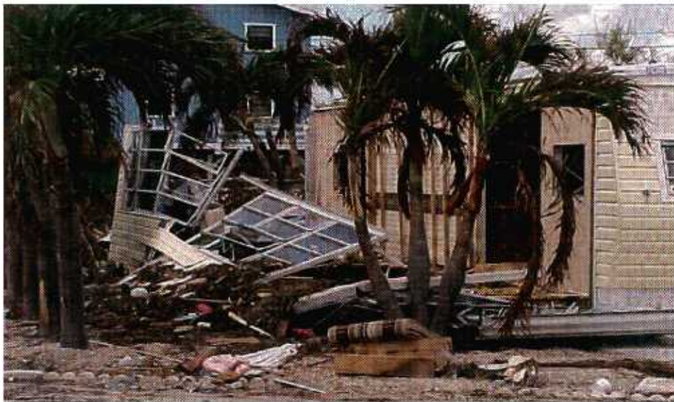
FIGURE 5-26 The addition to this manufactured home was destroyed, causing considerable damage to the rest of the home.
