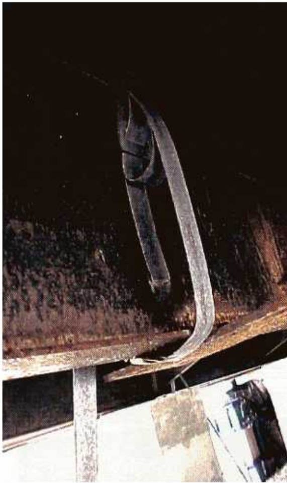
FIGURE 5-25 Proper strap installation.
