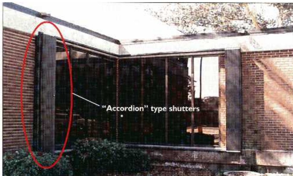
FIGURE 5-16 Window shutters on the Escambia County Administration Building.
