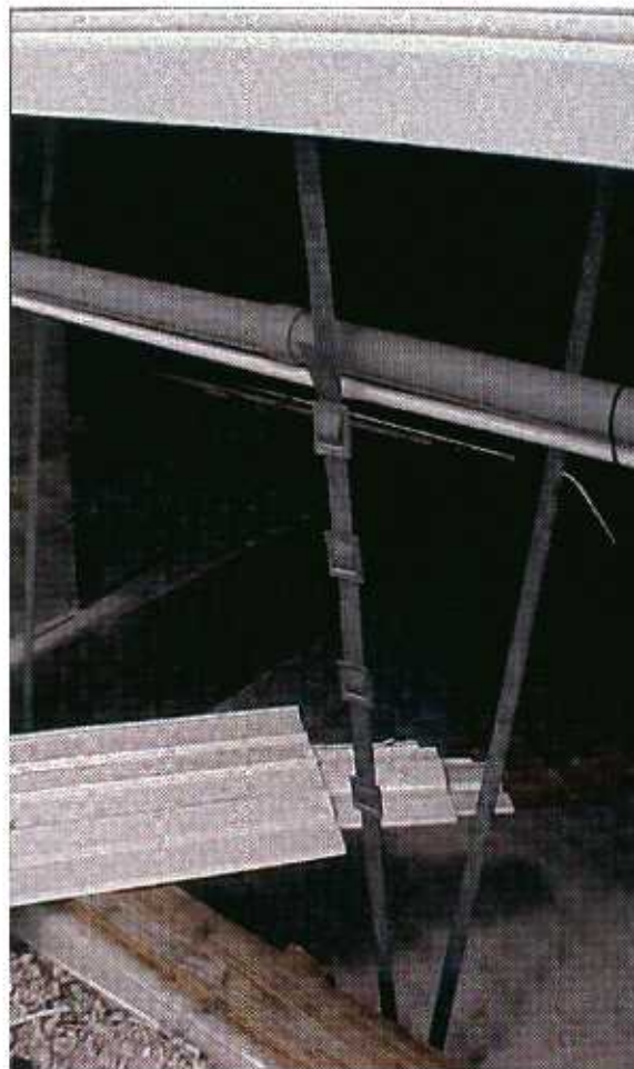
FIGURE 5-24 Improper strap installation. The buckle should be positioned where the strap wraps around the beam as shown in Figure 5-25.
