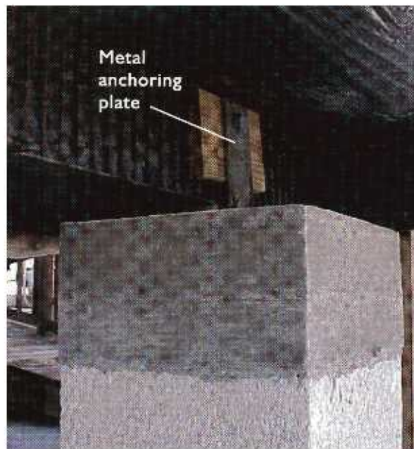
FIGURE 5-19 Reinforced masonry pier with metal anchoring plate.
