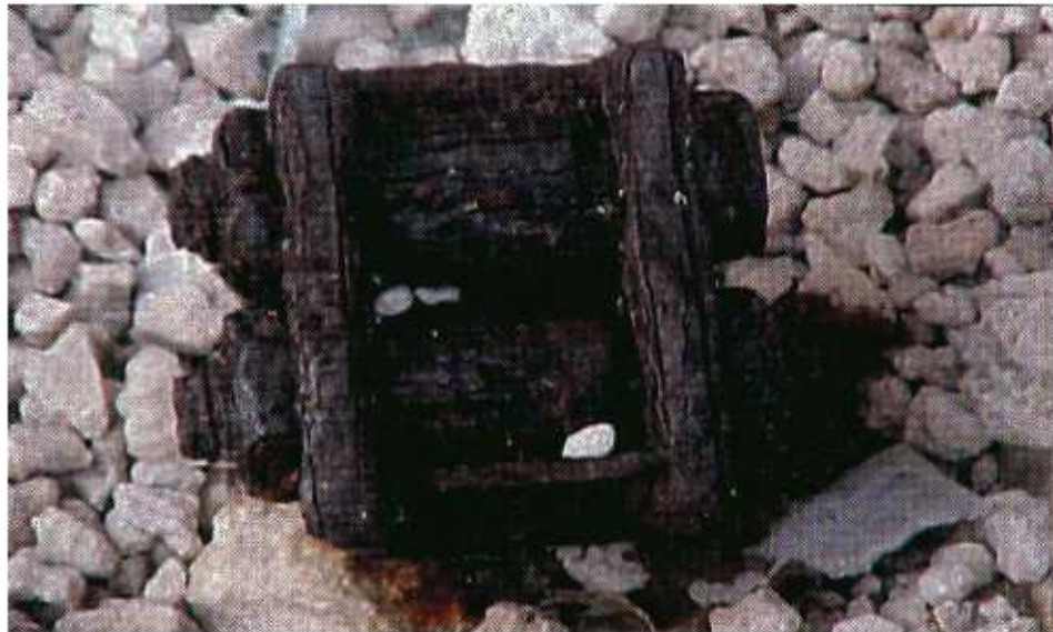
FIGURE 5-23 Rusted anchor under an older manufactured home. The State of Florida mandated galvanized anchors after January 1, 1999.
