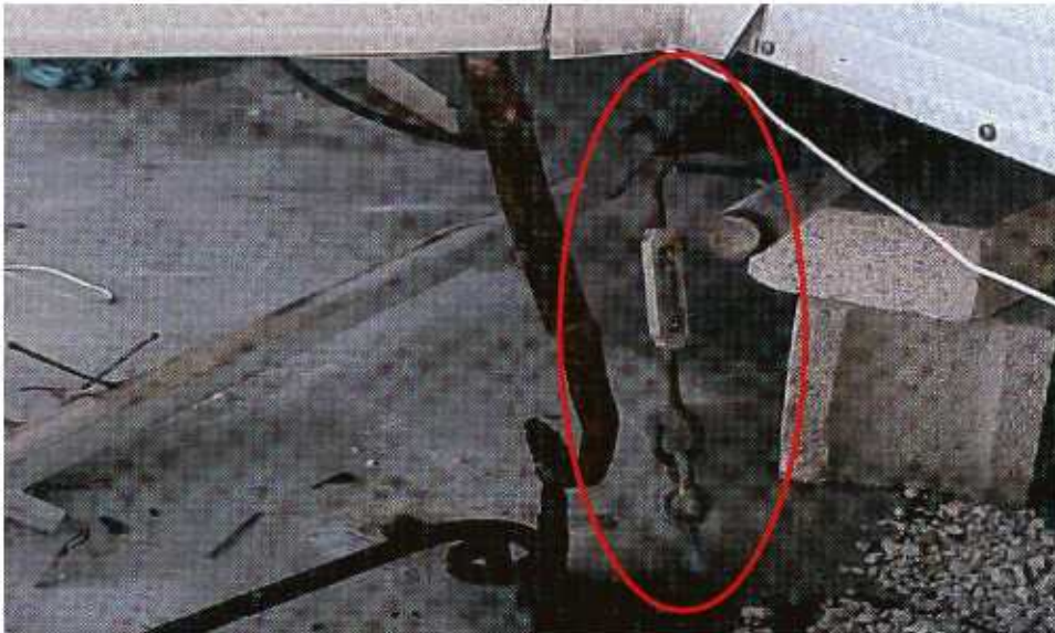
FIGURE 5-22 Inadequate turnbuckle anchor installed by homeowner on this older manufactured home. The home was severely damaged due to the lack of elevation, an unreinforced foundation system, and poor anchoring.
