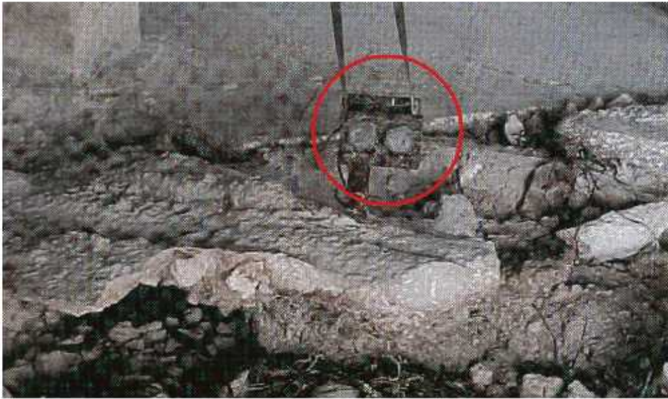
FIGURE 5-21 This anchor is only encased on the edge of the concrete fill pad and could easily be dislodged when the home is subjected to more severe wind or flood loads.
