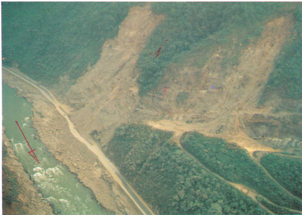
This Jogimara Rockslide repeatedly occurred this year. At the right side is seen the lime stone quarrying. Similar rockslide occurred at the same place in August 1992 pushing a long distance bus into the Trisuli River. The bus with all 28 passengers has not been found yet.
