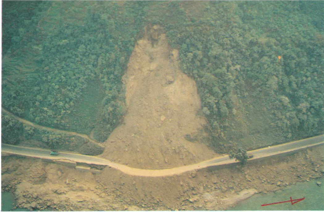
Another landslide near Jogimara
