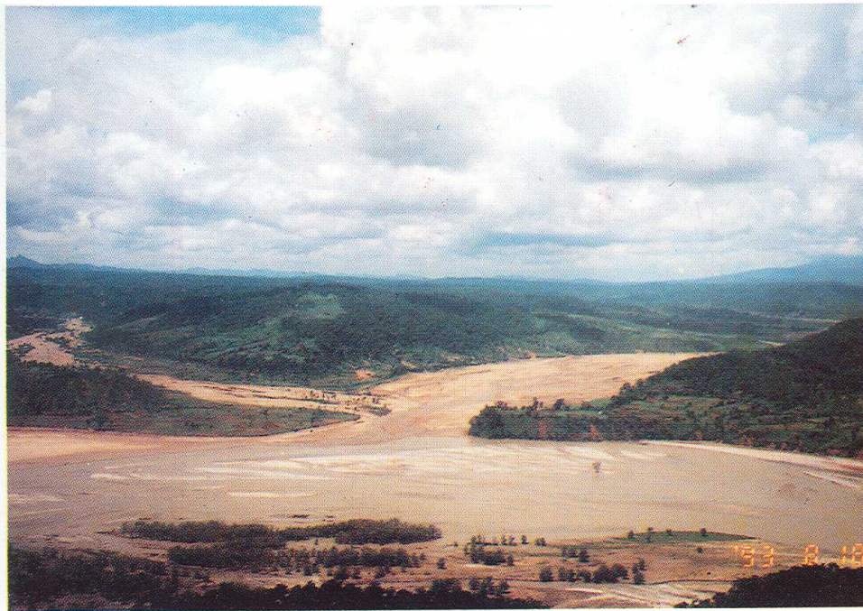
Bagmati River in the upstream of Barrage. Heavy siltation from tributaries of Inner Terai.
