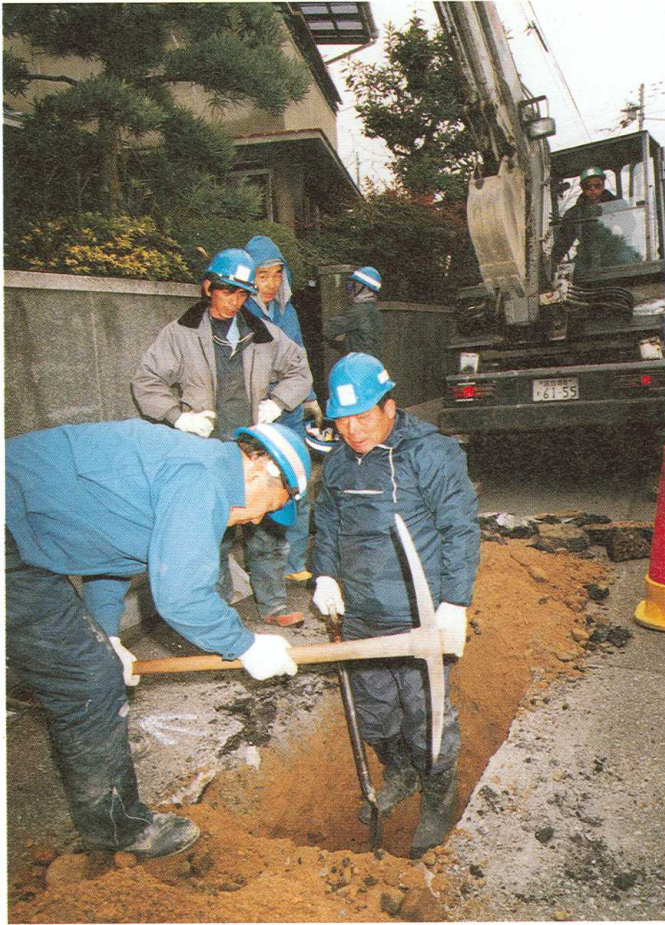
▲ Inspections of gas pipes. Gas supplies to 857,000 households were suspended immediately after the quake but were restored by April 20 except to vacant houses. It took three months to restore the gas supply system in order not to cause secondary disasters by gas leak.
