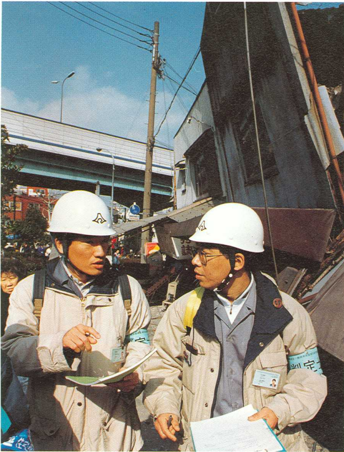
▲ Officials checking whether it is safe to enter damaged structures. © THE KOBE SHIMBUN
