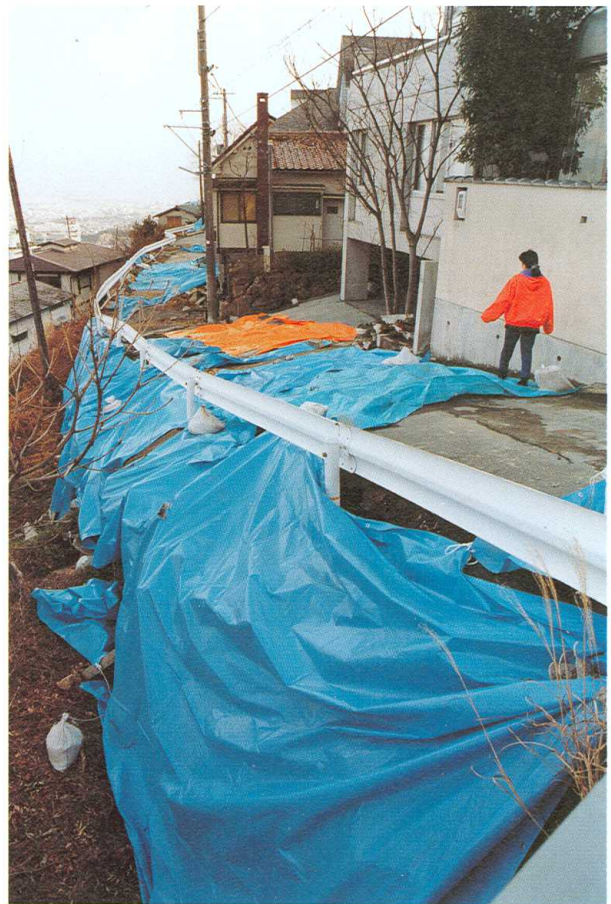
▲ Emergency measures taken at a place where a landslide was feared.
