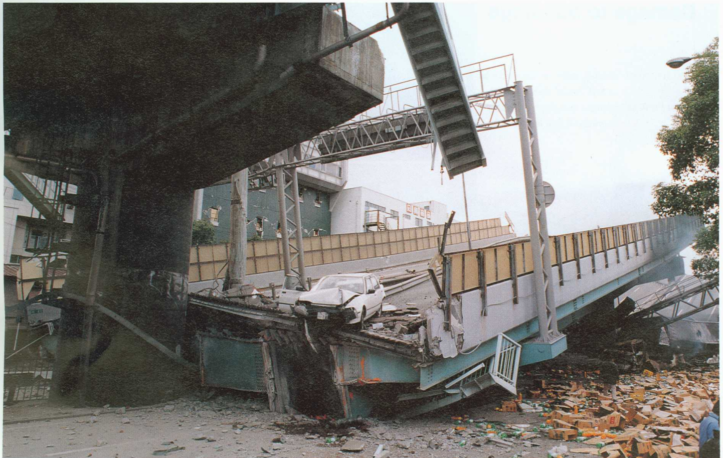
▲ An elevated bridge whose girder was dislocated.
