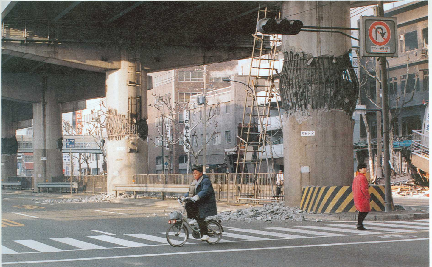
▲ A buckled bridge pier of an elevated road.
