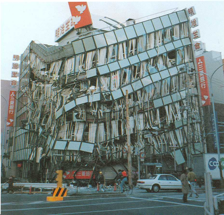
◀ A damaged building.
