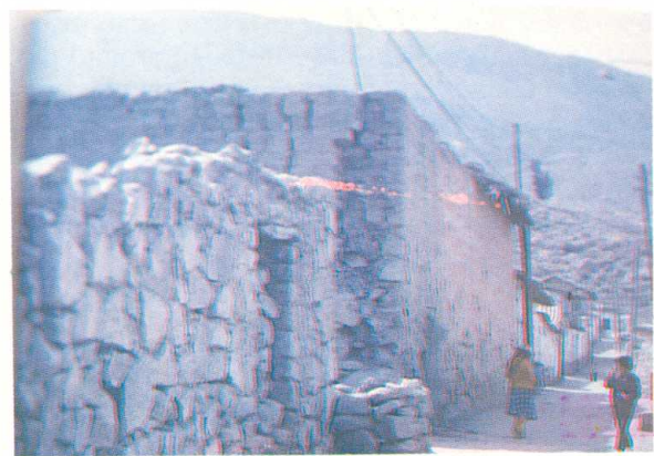
ADOBE CONSTRUCTIONS WEAKENED BY PAST EARTHQUAKES AND THE SOIL MOISTURE, WHICH INCREASES SEISMIC INTENSITY, MAKING THEM HIGH-HAZARD FACTORS. THE HIGH ADOBE WALL IN THE PHOTOGRAPH, SEPARATED FROM THE OTHER WALLS BY CRACKS, IS A HAZARD FOR PASSER-BYS.
