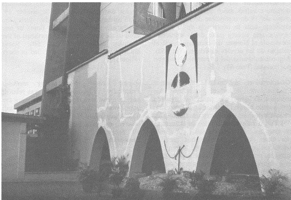
Photo 58.- RC "macroframes". Repair of the main entrance arches can be observed.
