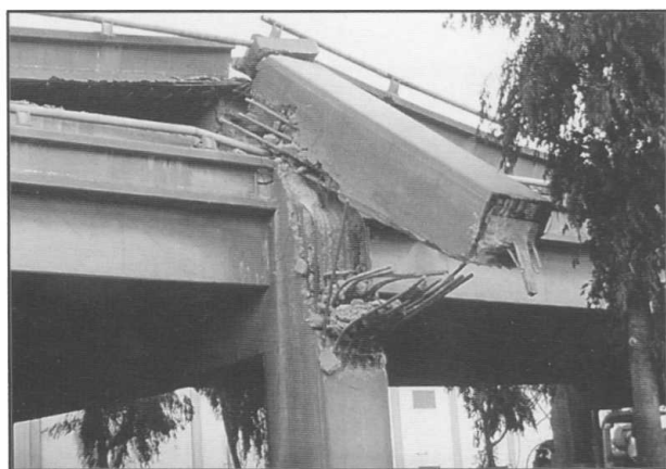
■ Figure 1 The collapse of the Cypress Street Viaduct in Oakland during the Loma Prieta earthquake of October 1989 was a major factor in the AASHTO decision to review the seismic design requirements in the Standard Specifications for Highway Bridges.
