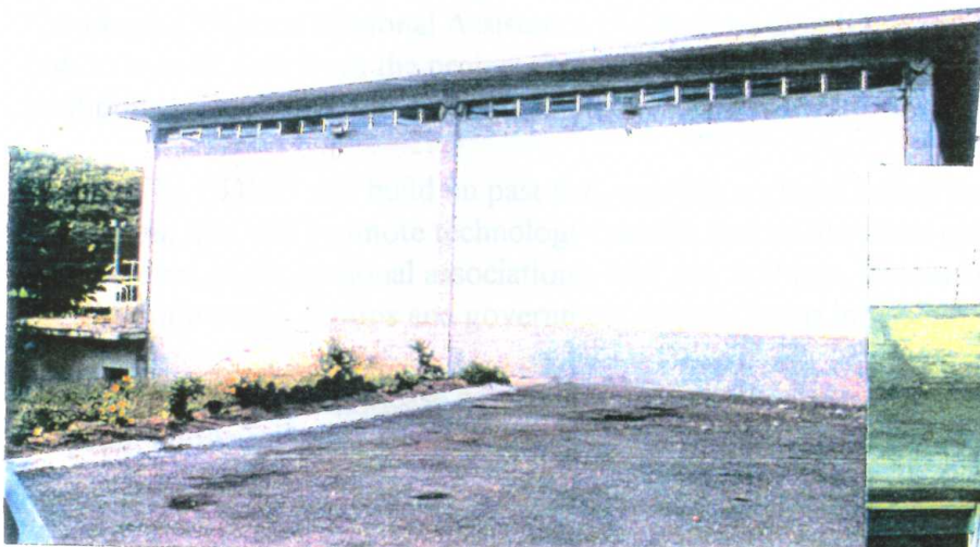
Figure 5: Building Housing Water Treatment Plant in Kingston. Walls on Exterior Restrain Columns and Cause "Short Column" Effect. Inset Shows Damage to Centre Column. [Woodford (Jamaica) Earthquake].
