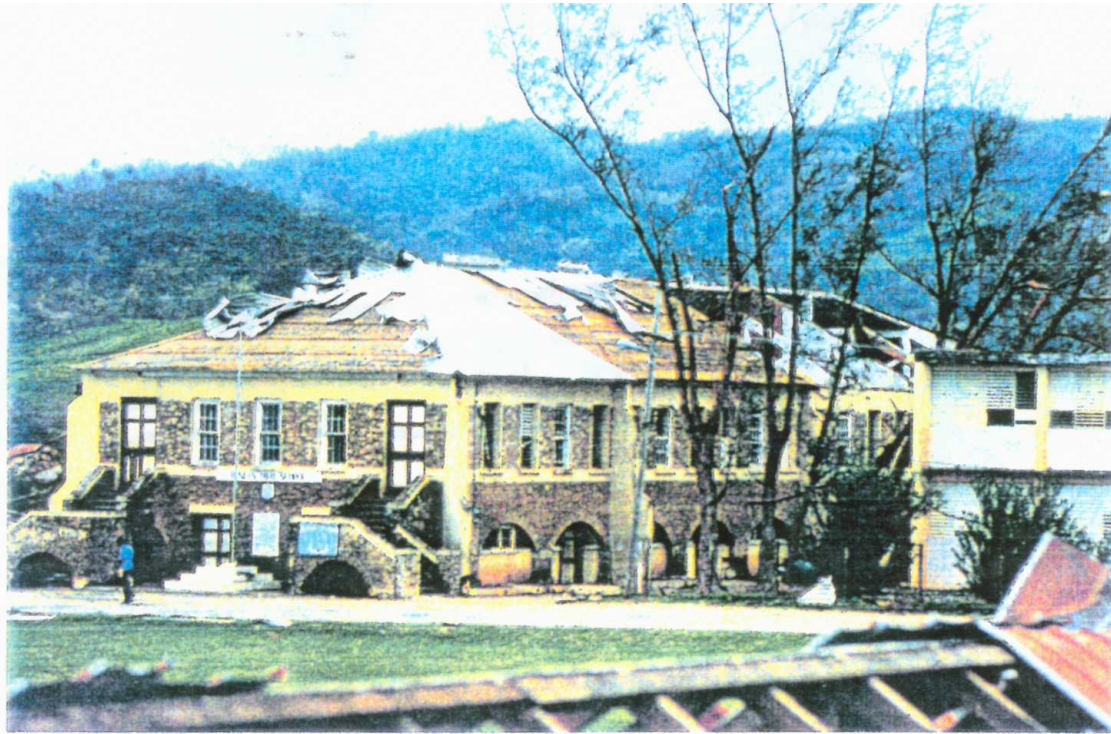
Figure 2: Hurricane Gilbert (1988) - Damage to Roof of Classroom Block at Ruseas High School in Luvea (N.Coast, Jamaica)
