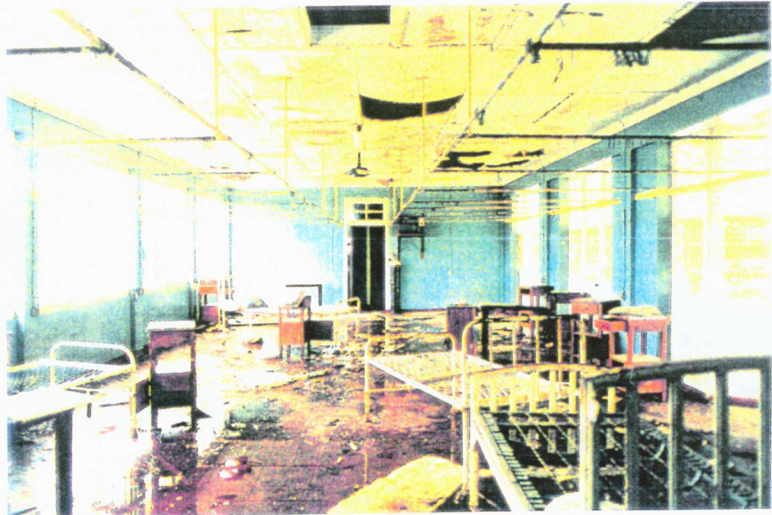
Figure 3: Interior Damage to Male Ward of the Noel Holmes Hospital Caused by Loss of Roof Sheetting - Hurricane Gilbert (1988)
