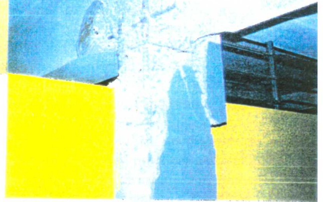
Figure 4: Above, Two Story Classroom/Library Building at Jamaica College, Kingston. Inset, shows Upper Level Column Damage Caused by Adjoining Wall Restraint. [Woodford (Jamaica) Earthquake].
