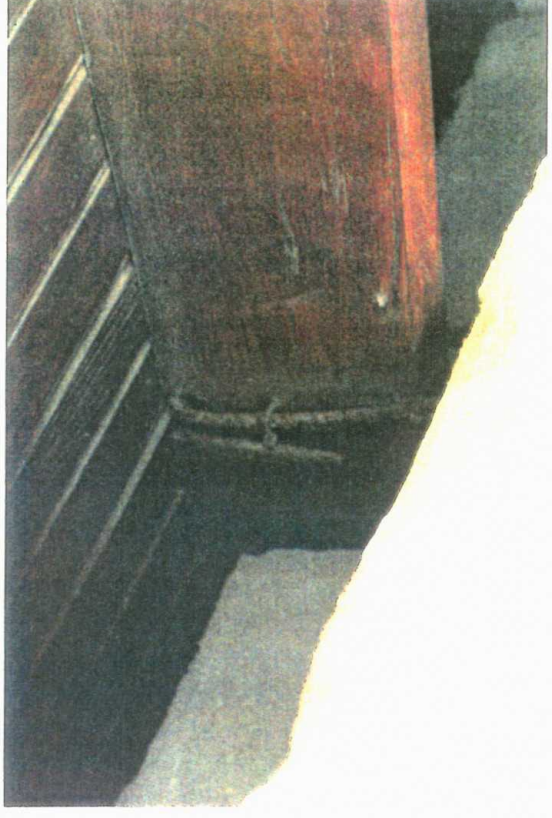
Photo 4: Rafter/beam connection, Administrative Offices atrium roof
