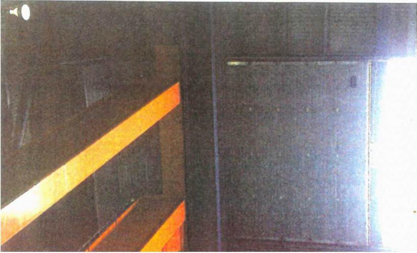
Photo 20: Roller shutter, Power Station
