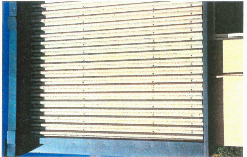
Photo 49: Typical side cladding detail, Garage
