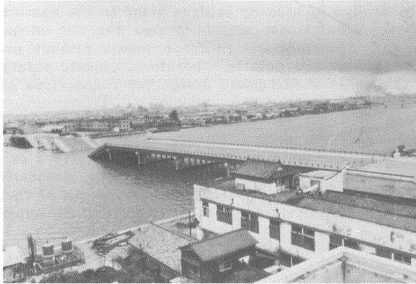
Photo 2 Damage of Showa Bridge by the Niigata Earthquake of 1964
