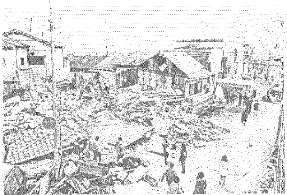
Photo 4 Building Collapse in Suma-Ward Residential District Collapse of two story wooden housing Hyogo Prefectural Government
