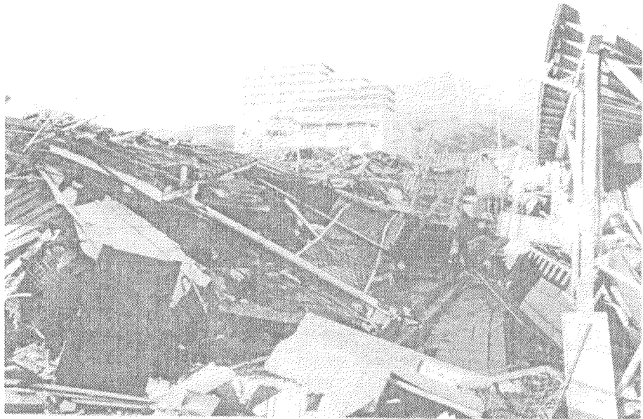
Photo 6 Collapsed Two Story "Bunka Apartment" In the back there is a SRC building with no damage Hyogo Prefectural Government
