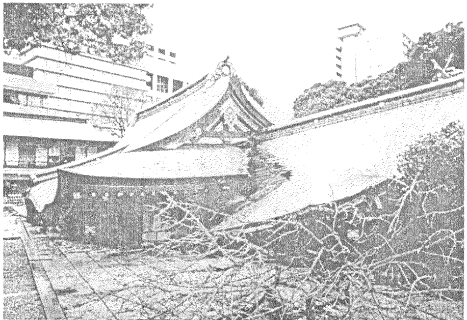
Photo 7 Traditional Wooden Column and Heavy Roof Shrine Collapsed In the back another undamaged SRC building Hyogo Prefectural Government
