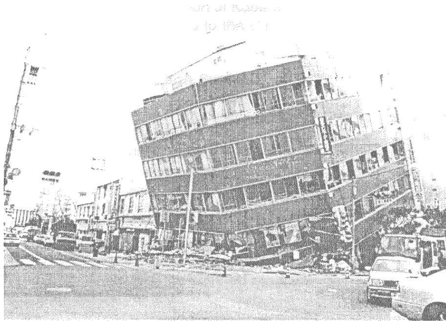
Photo 8 Ground Floor Collapse of Steel Structure Building Ground floor with not enough structural walls gave in Kobe Municipal Office
