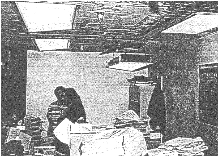
PHOTOGRAPH B7.5. Successful performance of two back-up support wires for fluorescent light fixture, Olive View Hospital. At this facility, this good performance was common and the failure shown in PHOTOGRAPH B7.4 was rare photo credit Bob Reitherman, Earthquake Engineering Research Institute
