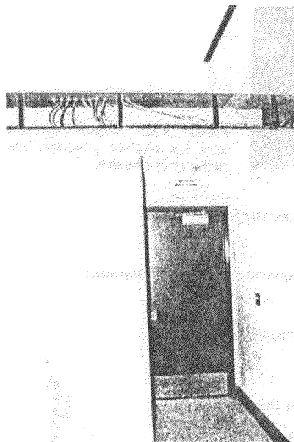
FIGURE 3.31 All wiring should be installed with slack. Shown here is wiring with proper slack, as well as wiring that has been pulled tight.
