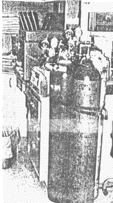
FIGURE 3.96 Unsecured gas cylinders such as these could be dangerous to both life and property during an earthquake.
