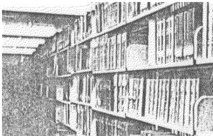
FIGURE 3.140. These bookshelves have been anchored to the floor and have lateral bracing in the longitudinal direction. They lack top bracing and shelf parapeets.
