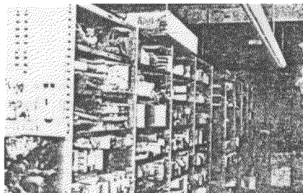
FIGURE 3.147. General storage shelves such as those shown here require base anchorage, longitudinal bracing, top bracing, and shelf parapeets. This shelving unit has not received any of this protection.
