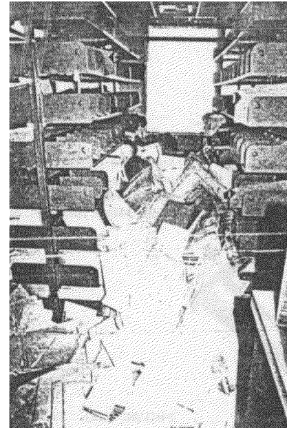
FIGURE 3.191. Spilled files such as these can be prevented by shelf retainers. Photograph courtesy of J. R. Harris, National Bureau of Standards.
