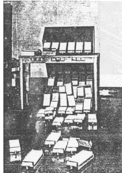
FIGURE 3.196. Even items such as library card files pose a potential threat to personnel. Photograph courtesy of Richard Miller and the National Science Foundation
