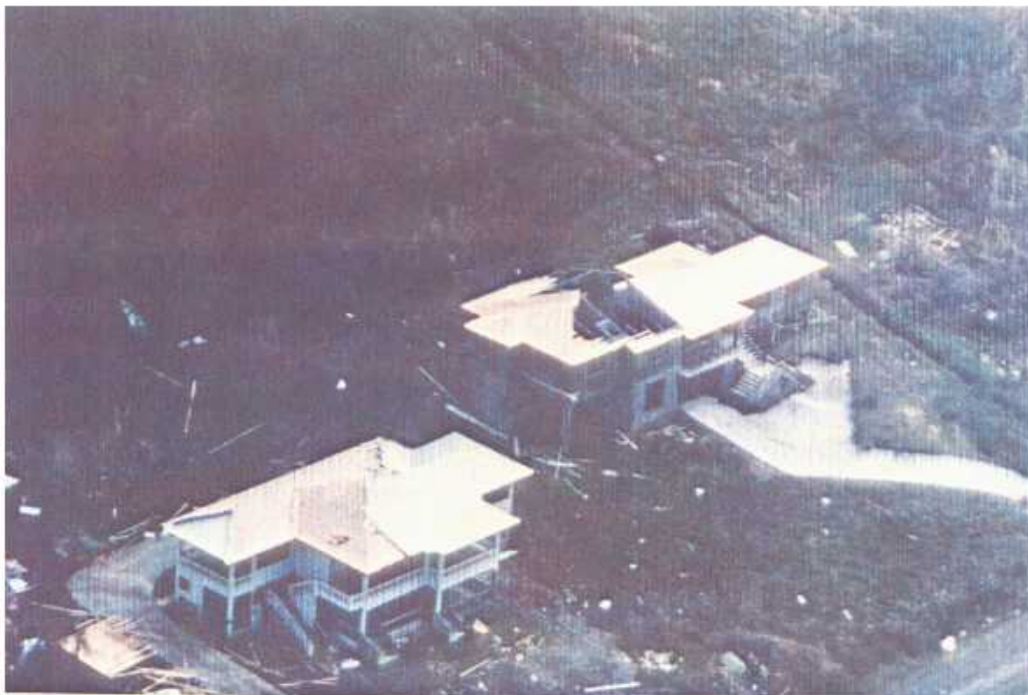
PLATE 25. Upper Income Houses. Note loss of some roof cladding to one house.
