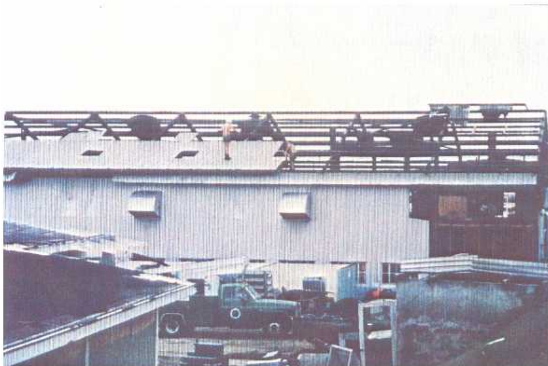
PLATE 28. Monlec Power Station. Loss of corrugated roof sheeting. The mechanism for fixing corrugated roof sheets must be carefully detailed and installed as per the Guidelines.
