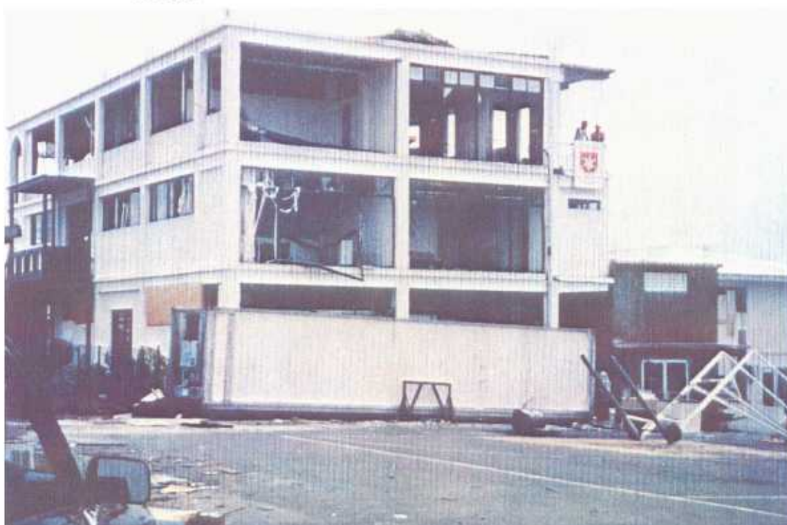
PLATE 26. Concrete roof. All windows and glass panels blown out or broken by flying objects.
