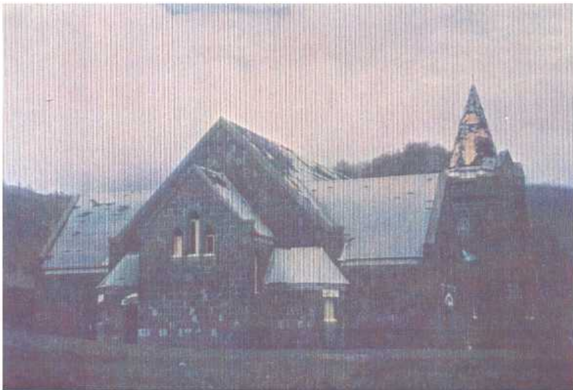
PLATE 38. Bethel Church. Church with traditional construction. Note loss of some shingles on the spire, but the church was otherwise undamaged.
