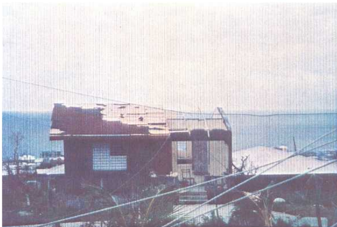
PLATE 29. Low income house at Webbs. Note failure of roof at gable and blown out wall.
