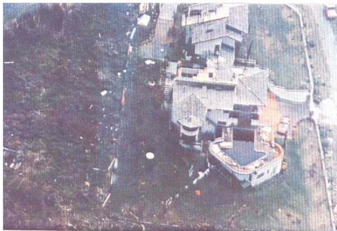
PLATE 24. Private large house with swimming pool. Some hipped roofs are intact, but shed type roofs lost their roof covering and some framing.
