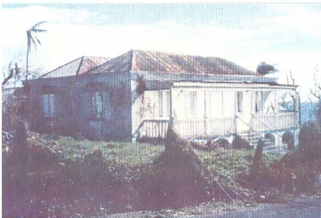
PLATE 34. Traditional middle income housing with good hurricane resistant features. Note hipped roofs of high pitch and no overhangs. Note also that the verandah to the house in Plate 21 has a separate roof. These houses have permanent timber hurricane shutters.
