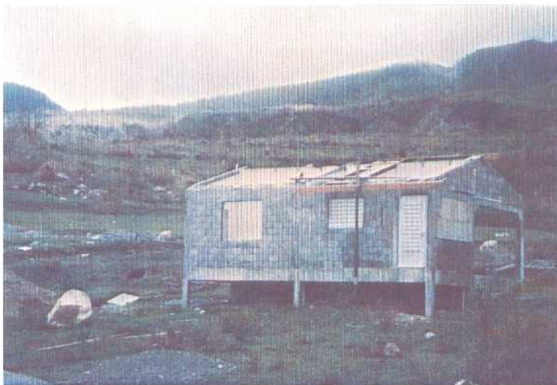
PLATE 31. Low income house on concrete posts and concrete cill-beam. The frame of the house appeared to be well constructed, but the low roof pitch on inadequate holding down details led to the loss of the roof.
