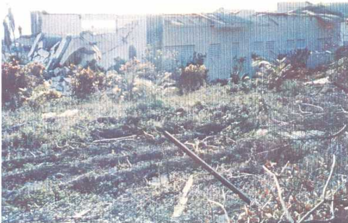
PLATE 37. Collapsed masonry walls. Loss of roof structure and cladding. Church in Plymouth allocated as a hurricane shelter. Poor construction led to complete loss of roof and collapse of the masonry walls. Buildings to be used as shelters should be designed to be hurricane and earthquake resistant and must have appropriate facilities.
