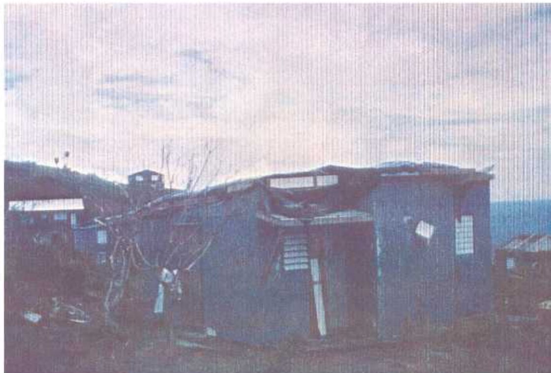
PLATE 30. Low income house at Broderick. The low pitched shed roof was lost. Such roofs are very vulnerable to high winds.
