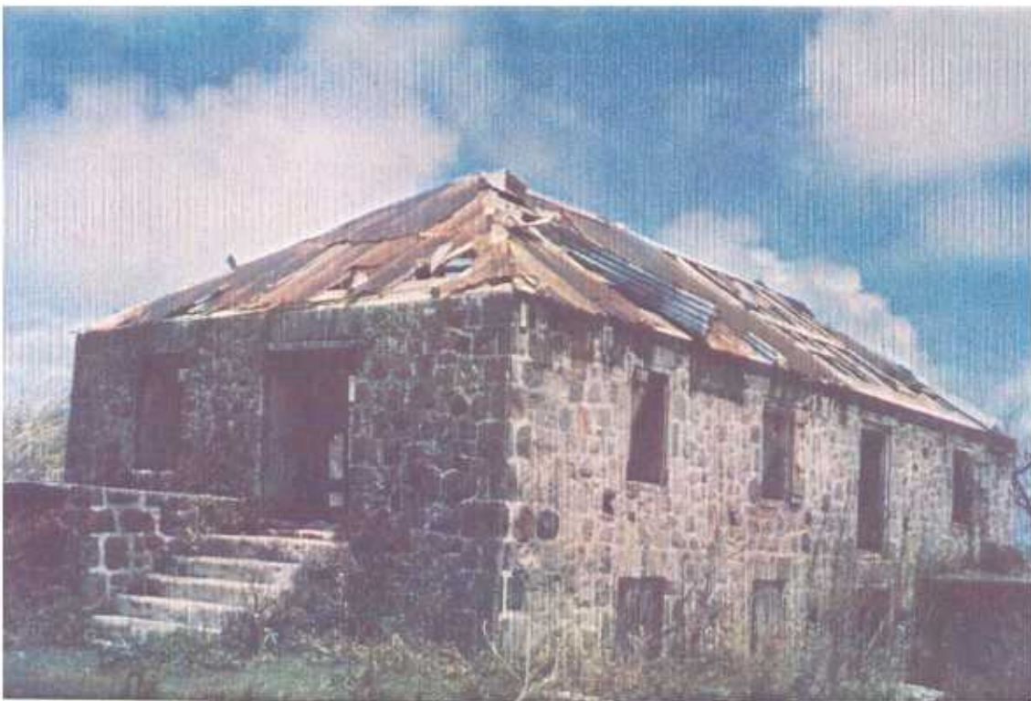
PLATE 36. Abandoned building in poor condition. Although the galvanised iron sheets are badly corroded this building might have survived damage due to the excellent shape of the roof and traditionally strong construction details.
