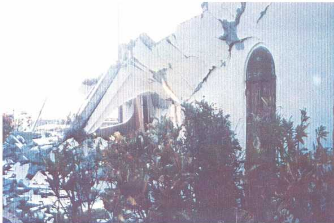
PLATE 40. Church in Plymouth. Collapse of unreinforced masonry walls.
