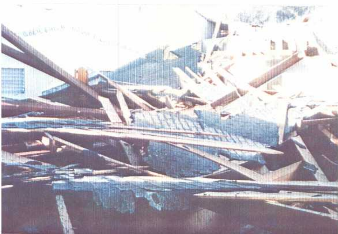
PLATE 39. Church in Plymouth. Collapse of roof structure.
