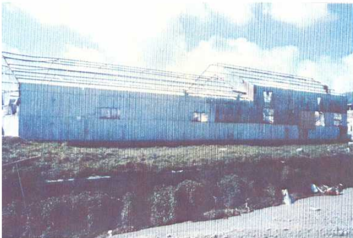
PLATE 27. Ginnery. Note total loss of corrugated roof sheeting . Steel roof frame in place but with some buckling of the purlins.
