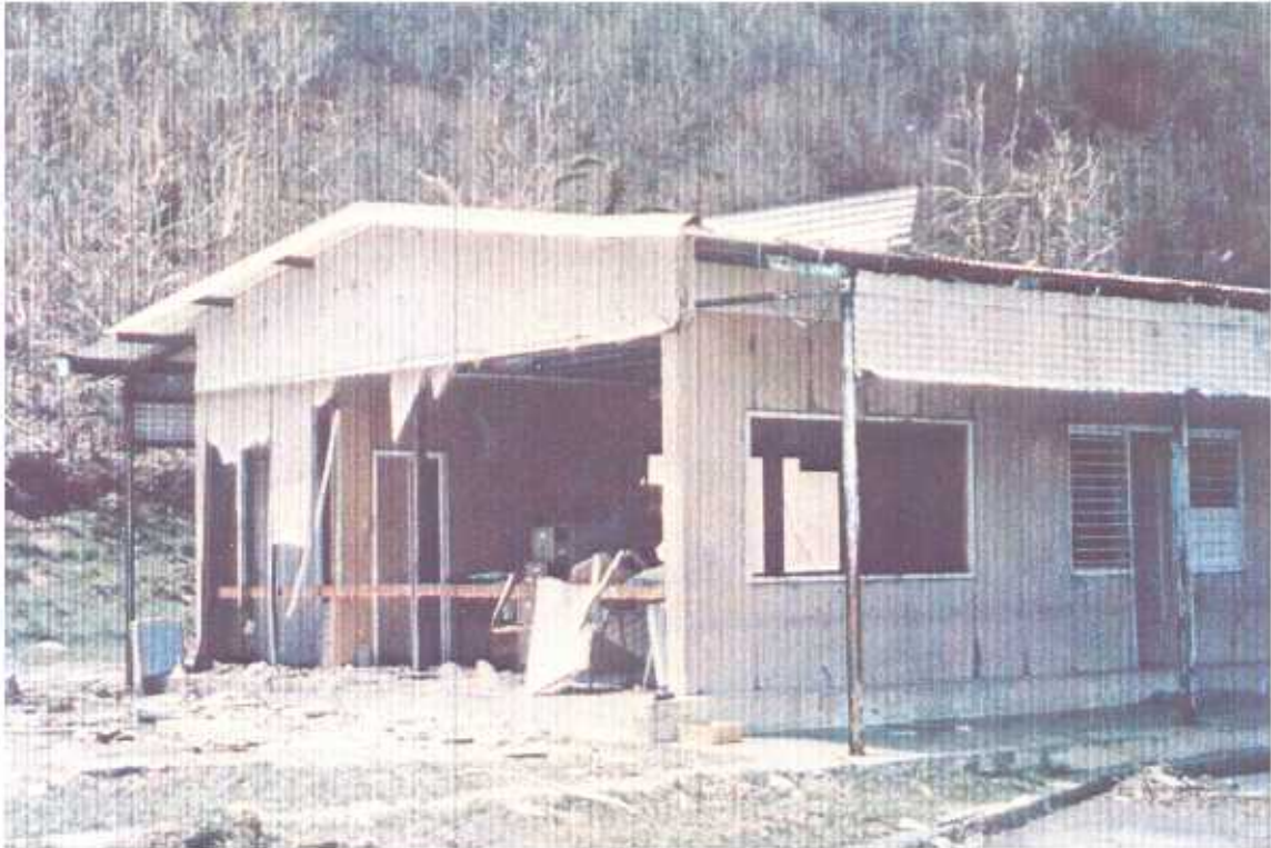
PLATE 45. Harris School. 60mm thick sandwich panel walls. Gable and walls, windows and doors blown in.
