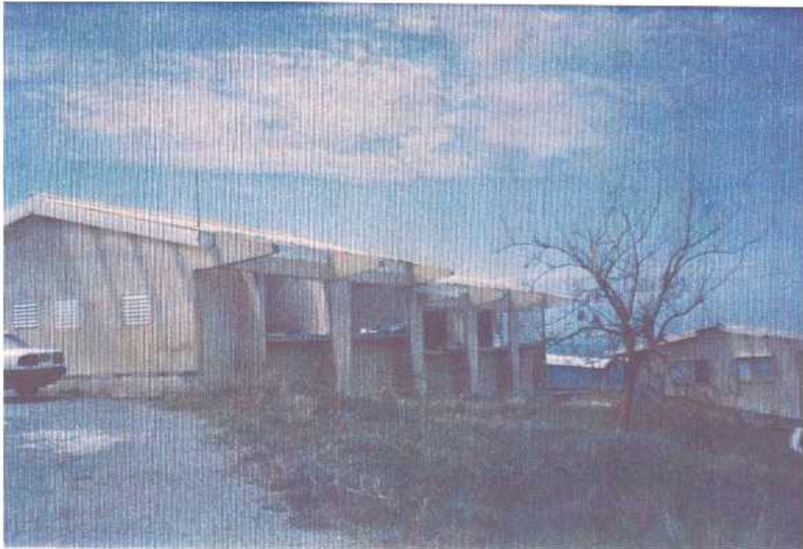
PLATE 51. Brades School. Sheeting loss from canopy roofs, windows blown out.
