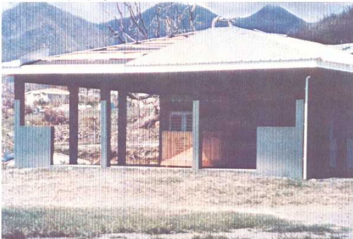
PLATE 46. Montserrat Secondary School. Loss of sheeting of hipped roof
