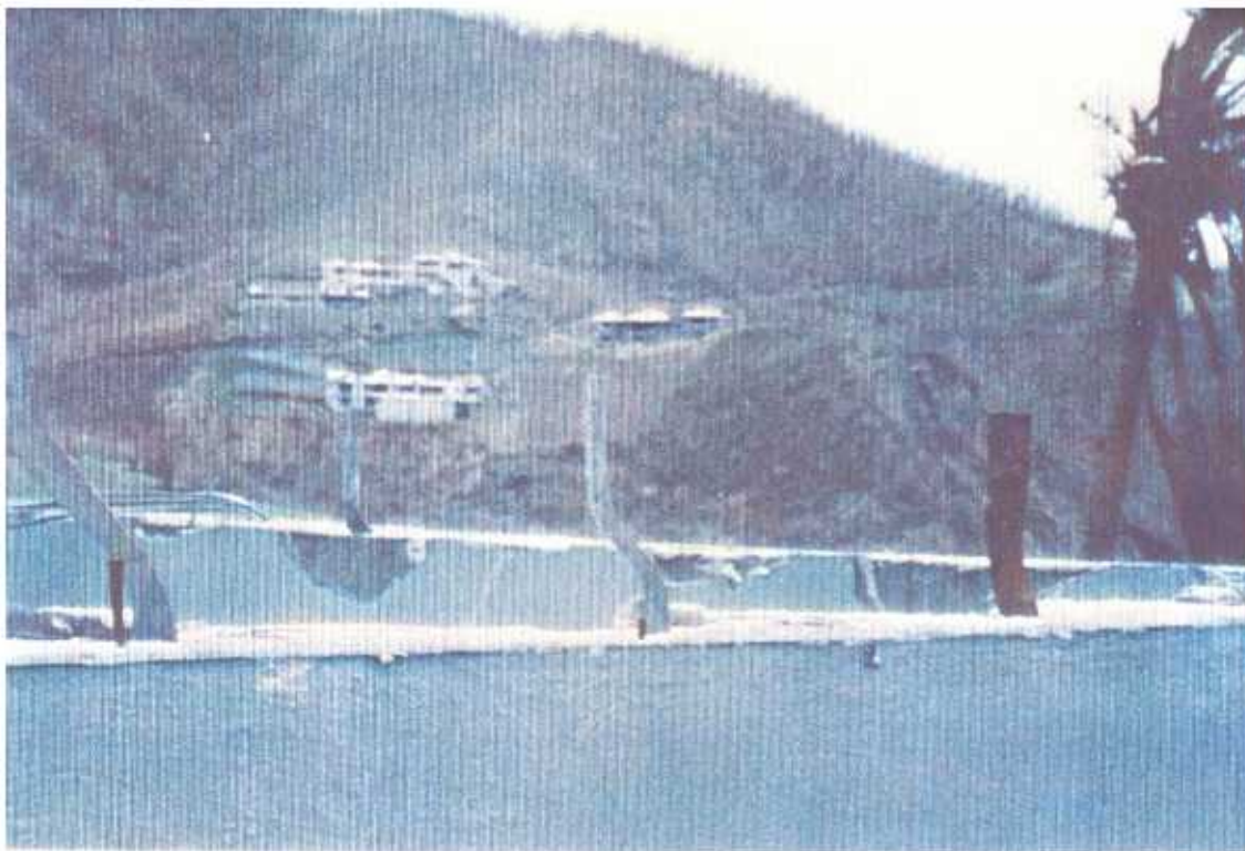
PLATE 59. View Pointe Hotel. Holding down straps, straightened out by uplift forces on unit that has lost its roof.
