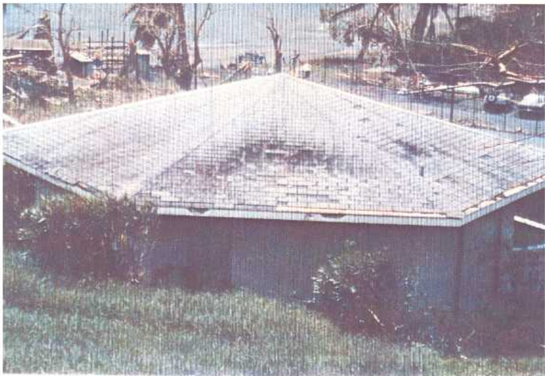
PLATE 58. View Pointe Hotel. Hipped roof performed with limited damage on hexagonal room units.
