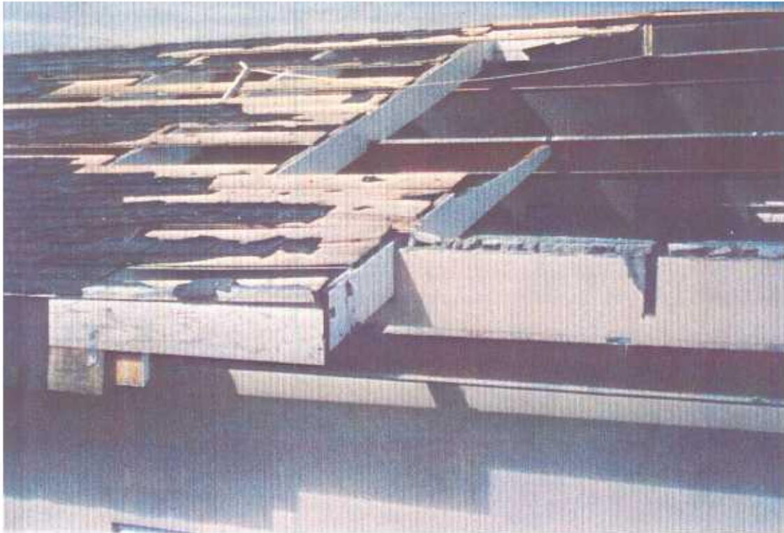
PLATE 49. Bethel School. Loss of roof cladding and rafters due to inadequate construction
