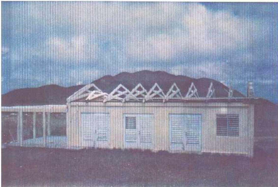
PLATE 50. St John's School. Complete loss of roof cladding from pitched roof and flat roof of open assembly area.
