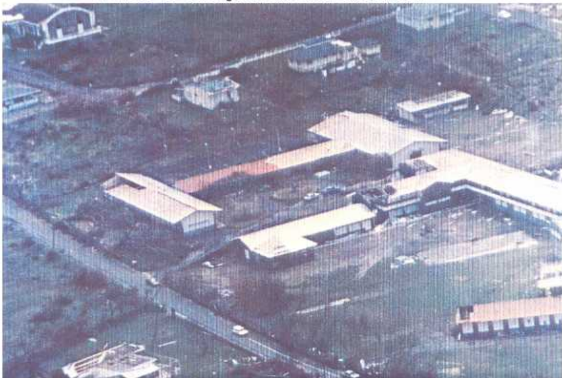
PLATE 42. Aerial view of Technical College and Secondary School. Note Typical roof failure at gable ends. Roof pitch too shallow for "normal" construction .
