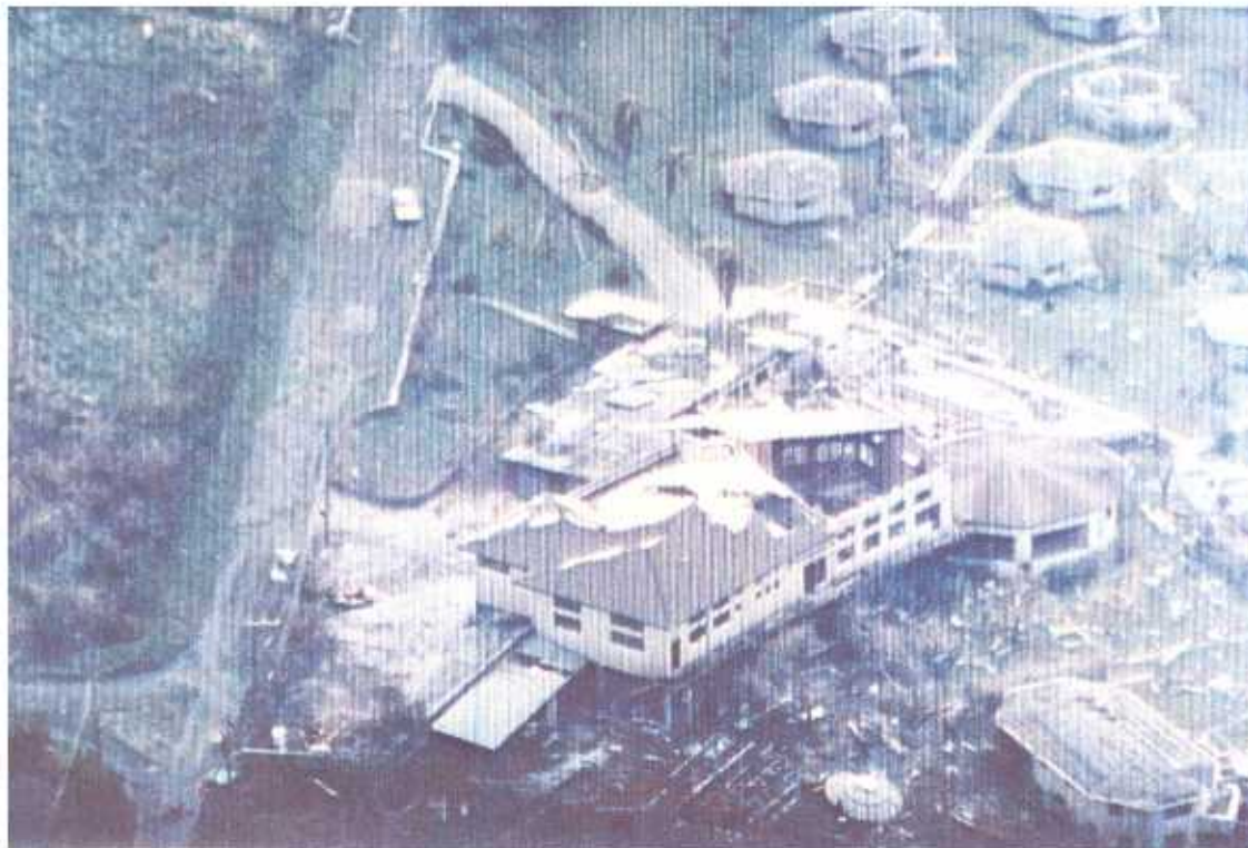
PLATE 56. View Point Hotel. Loss of roof cladding on flat pitched roof section.
