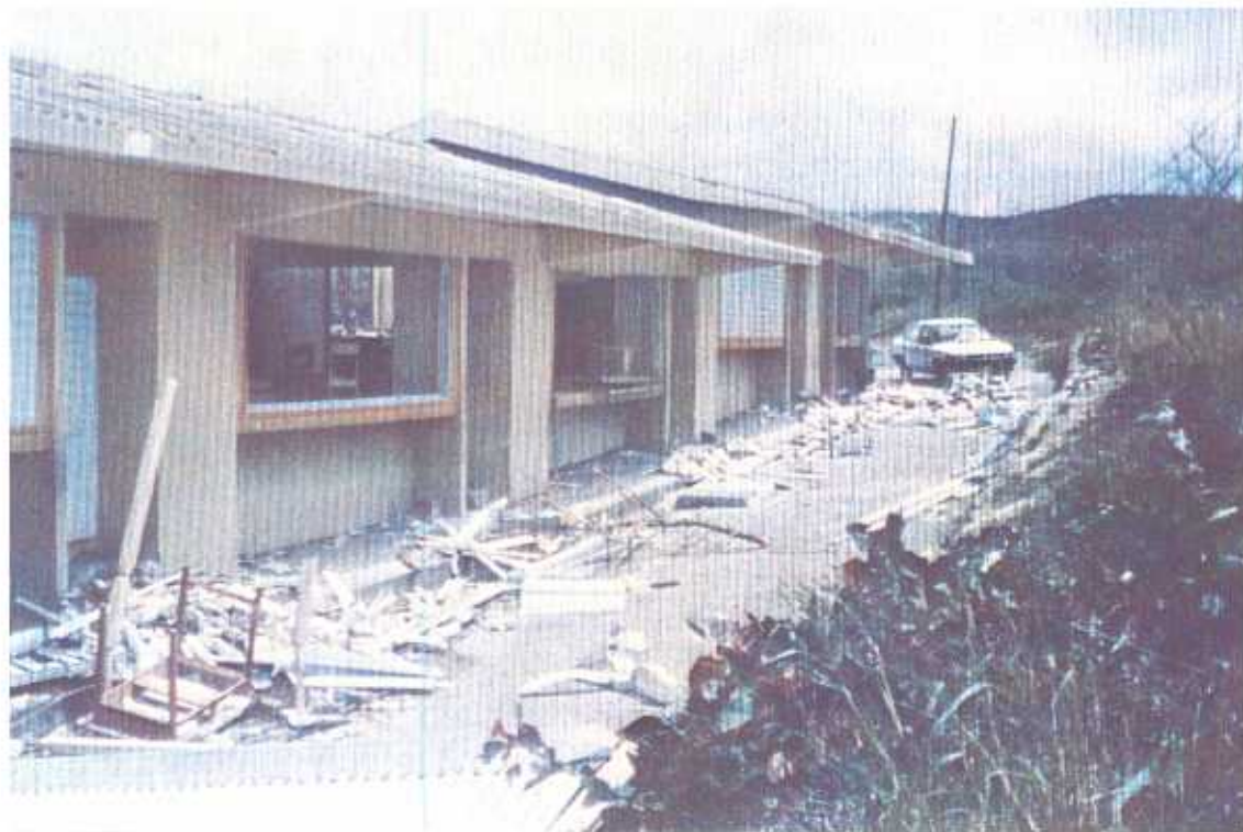
PLATE 52. Brades School. Large 12'x 5' aluminium louvre window blown out on both long elevations.
