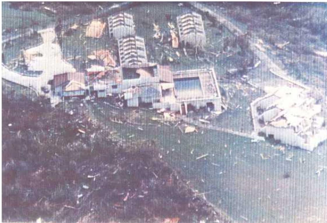
PLATE 55. Emerald Isle Hotel. General loss of roof. Note large sections of roofs on ground nearby. These gable ended roofs with shallow pitches are vulnerable.
