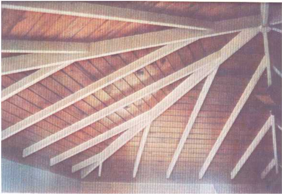
PLATE 57. View Pointe Hotel - Room Unit. An example of good roof framing. This level of construction must be maintained for all elements of the roof to ensure resistance to high winds.
