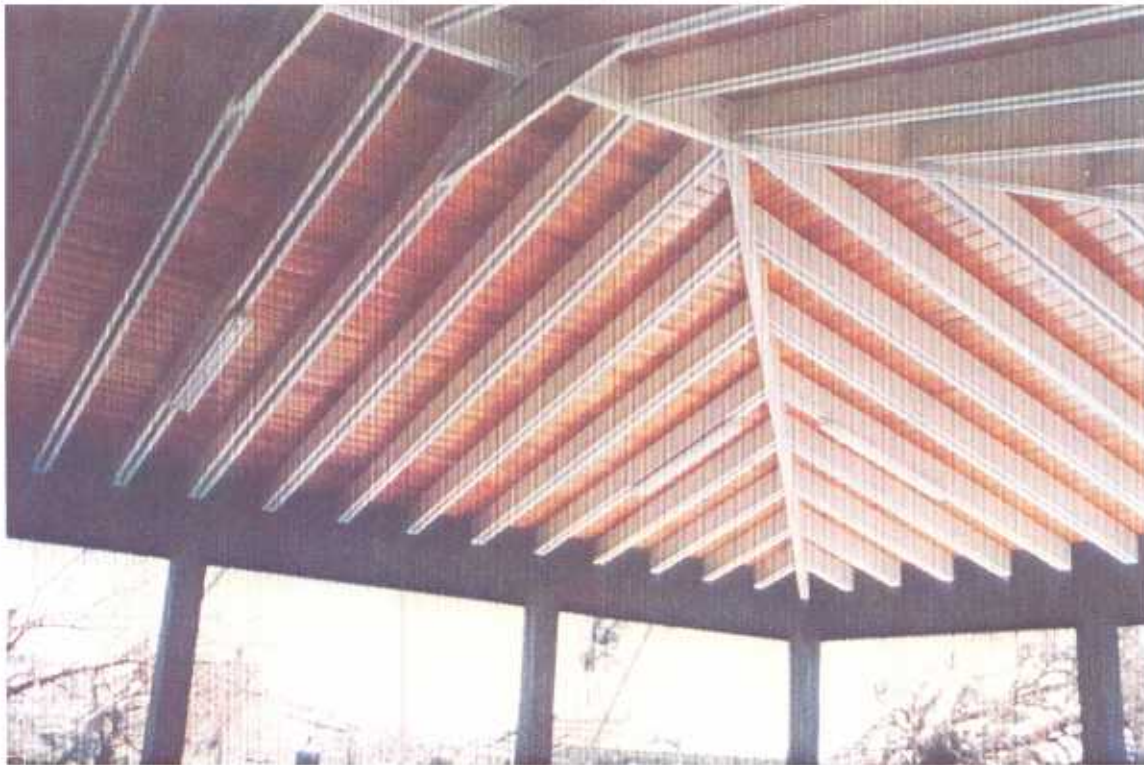
PLATE 43. Montserrat Secondary School. Well constructed hipped roof with close boarding. This roof performed satisfactorily.
