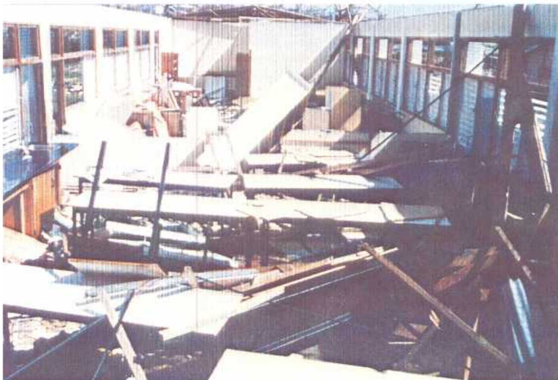
PLATE 44. The roof was completely destroyed and some windows blownout. Rebuilding to improved standards is necessary. (Chemistry Lab at Secondary School, Dagenham)
