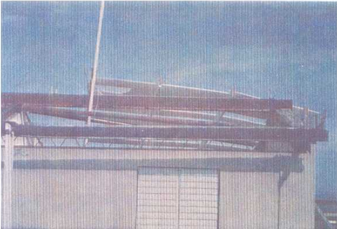
PLATE 47. Bethel School. Rafters failed at ridge joint.
