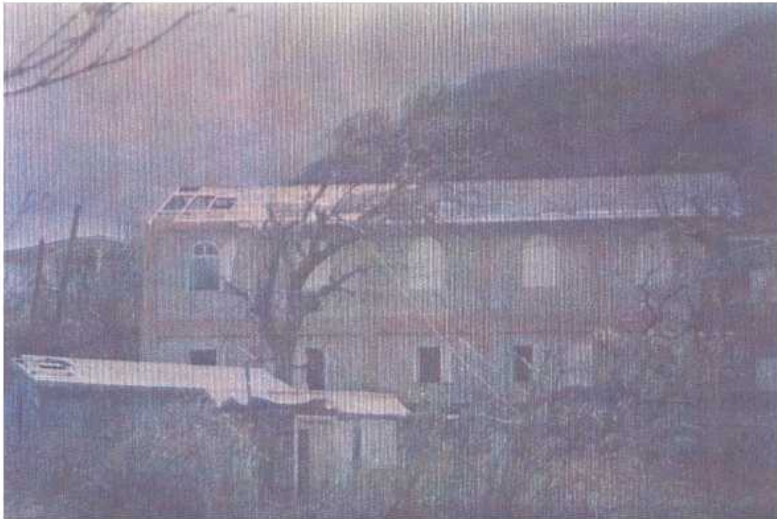
PLATE 41. Pentocostal Church - hurricane shelter. Low pitched roof, loss of sheeting at gable end.
