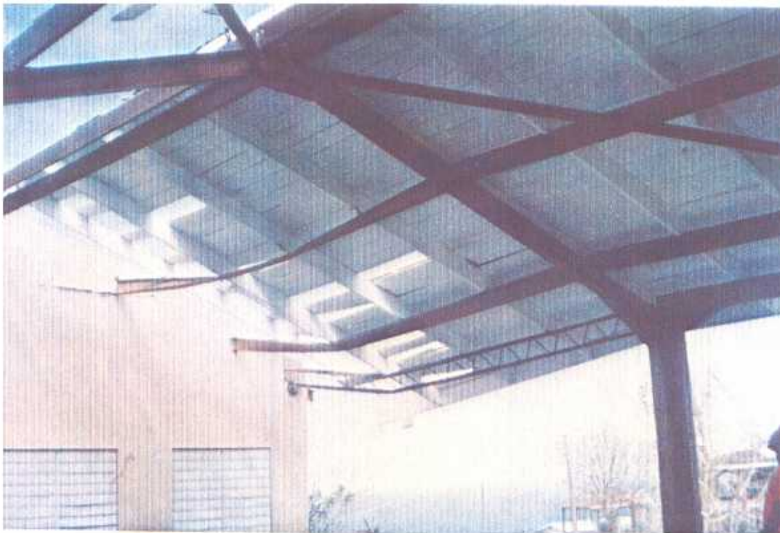
PLATE 48. Bethel School. Very inadequate roof framing contributed to the major damage.
