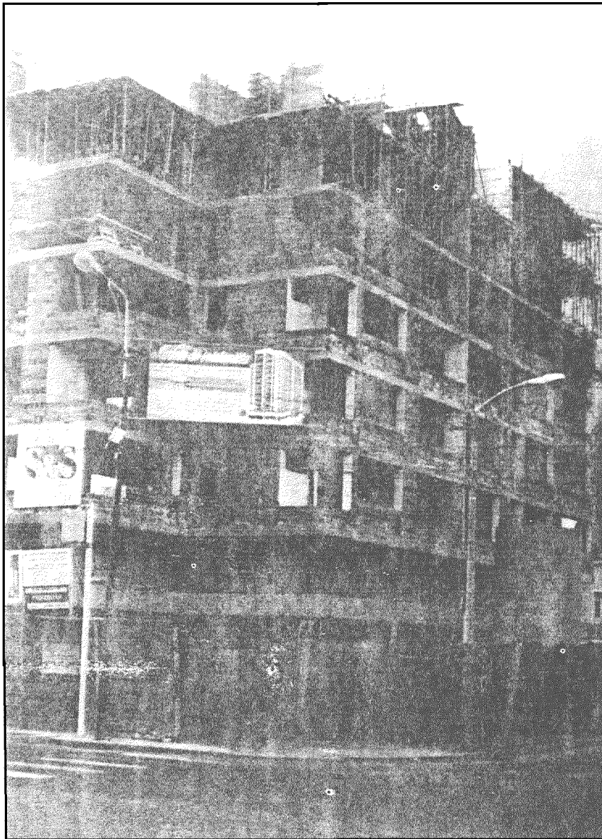
Multi-story building under construction in Bogotá, Colombia. This appears to be of a type of construction, common in many countries of Latin America, in which non-structural masonry walls and partitions are enclosed within a reinforced concrete structural frame. Although the integrity of this particular building cannot be assessed from a photo alone, the type of construction described is vulnerable to earthquake damage. (Photo by Oliver Davidson, Regional Preparedness Officer - Latin America and the Caribbean, US Office of Foreign Disaster Assistance.)
