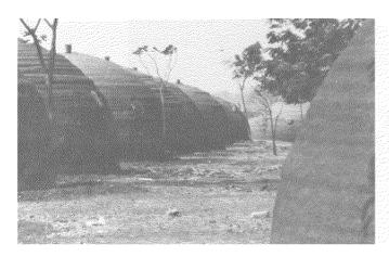
Adjacent to the E1 Coyotepe campsite in Masaya, Nicaragua, following the 1972 earthquake the West German Red Cross donated 500 polyurethane igloos. Although such units only take two hours to fabricate, it took 148 days for the first igloo to be occupied due to logistical problems as well as difficulty in obtaining a site with approval to build. Approximately 30 per cent of the igloos were occupied despite the fact that there were no rent charges.
