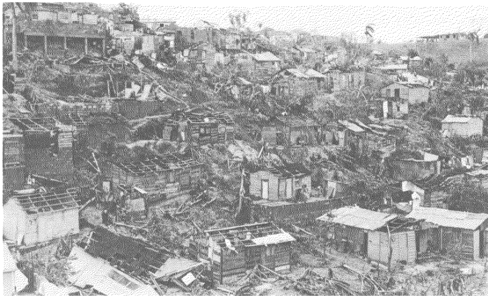
In areas subject to high winds, the roof is the most vulnerable part of the structure, as is indicated in this example after Hurricanes David and Frederick in the Dominican Republic, 1979. Improved building techniques can greatly reduce this risk.
