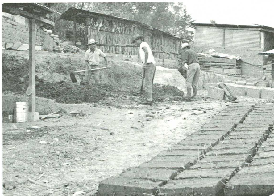
Men making adobe blocks to rebuild houses in Comalapa.
