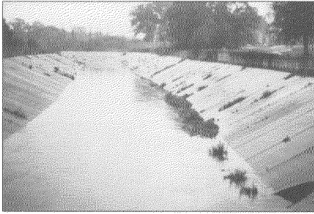
Storm drainage is a significant problem in many large urban areas, particularly if development has been rapid and not well planned. Drainage systems must be designed to handle infrequent, but potentially catastrophic, events.
