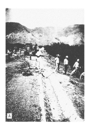
Figure 8. (A) View north along Highway CA-10 near Zacapa showing drainage ditch offset by 60-cm left-lateral and 5-cm south-side-down displacement on the Motagua fault, 8 February 1976. Black line drawn on north side of offset is alined with the upper inside edge of the section of ditch in the foreground.
