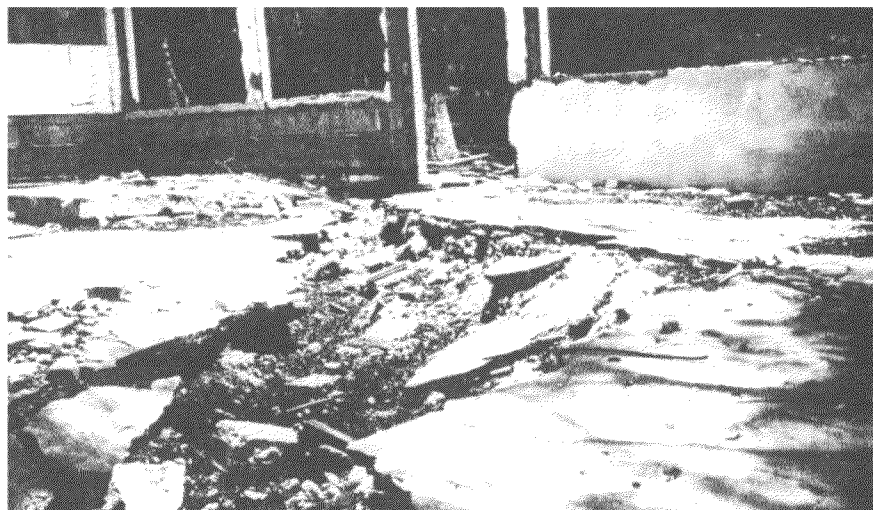
Figure 9. Floor of a concrete-block house pulled apart 1.5 m by lateral spreading. The house was located at the northwest end of the central lobe of the Villalobos River delta at La Playa.
